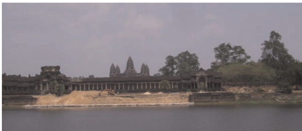
Figure 1. Intervention area during the rehabilitation intervention.
