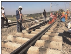
Figure 4. Removing rails.
