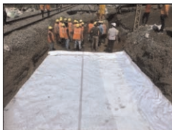
Figure 9. Laying the nonwoven geotextile.
