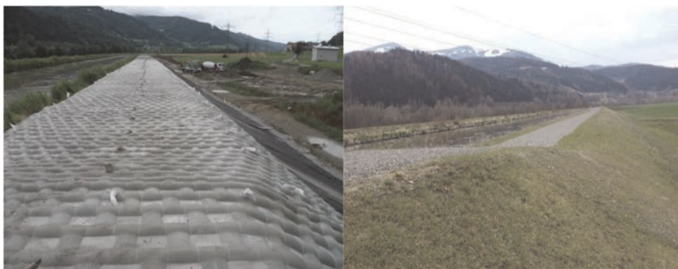
Figure 4. Concrete mattress: after installation (left); after being vegetated 2 years later (right).
