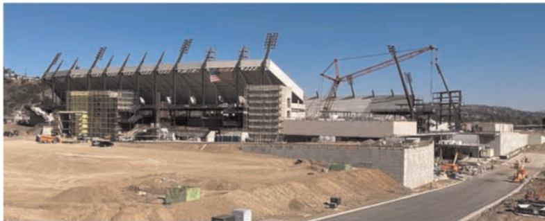
Figure 5. SDSU Stadium under construction.
