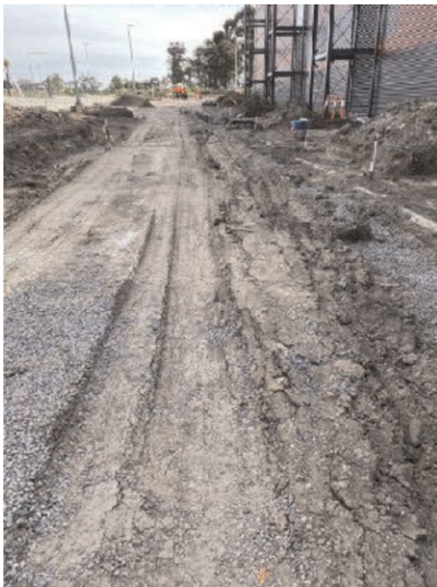
Figure 3. Installing crushed rock capping layer over geogrid.
