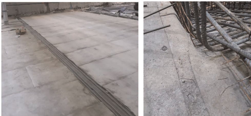
Figure 3. Geocomposite installed on the PVC geomembrane in Paris Line 16.
