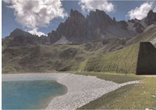
Figure 4. Avalanche protection dam Axamer Lizum after completion.
