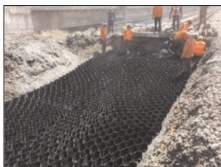
Figure 12. Bottom-most geocell layer.
