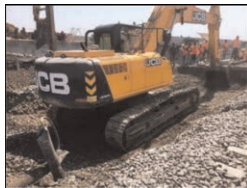
Figure 5. Removal of sleepers.
