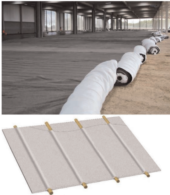
Figure 2. Installation of the geocomposite on the subgrade.
