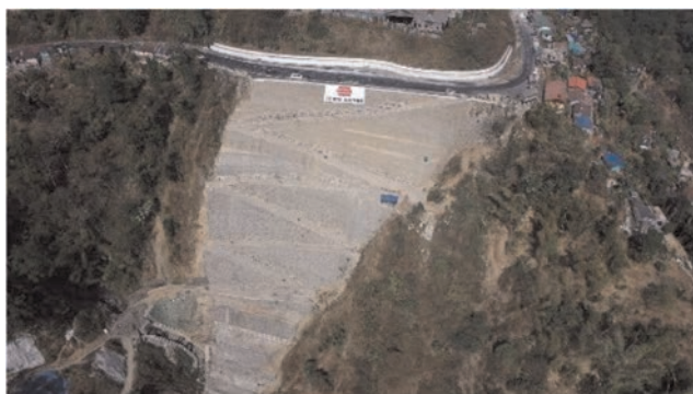
Figure 15. The completed structure.
