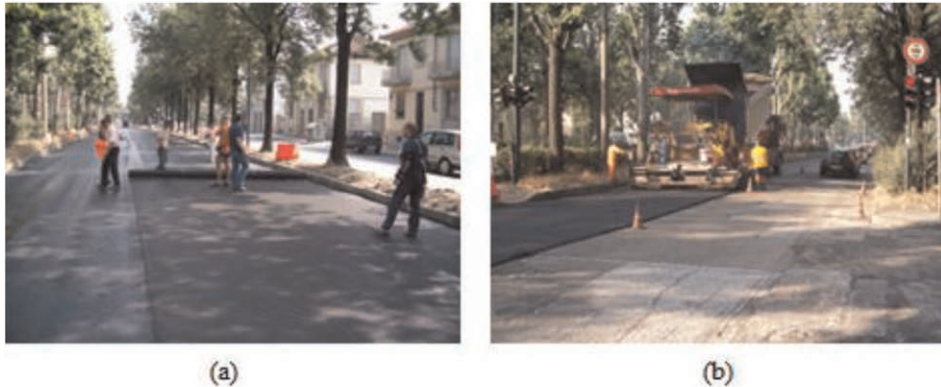
Figure 1. Installation of the HaTelit C 40/17 asphalt reinforcement (a) and asphalt placement on unreinforced section (b) (June 2005).
