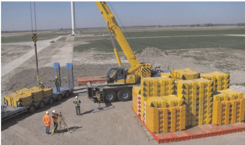
Figure 3. Wieringemier project – general view of the full-scale test.
