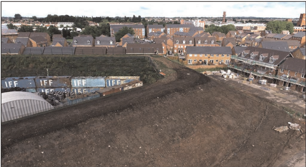
Figure 4. Aerial shot of the completed bund.
