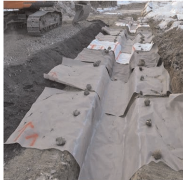
Figure 5. Installed geotextile samples.
