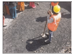
Figure 11. Compaction with manual hand tamper.
