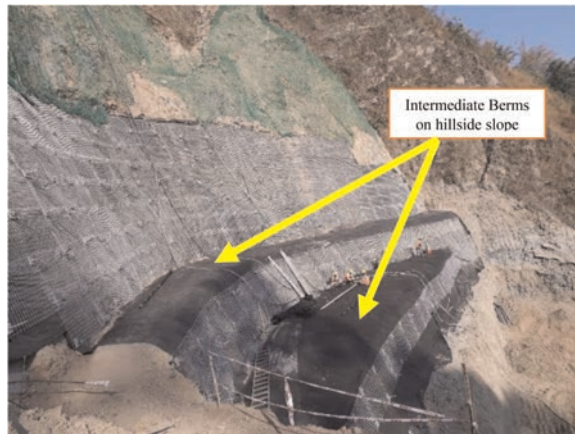
Figure 14. Slope stabilization through installation of soil nails and fixing one layer each of non-woven geotextile and GI back mesh.
