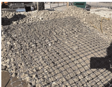
Figure 2. Close-up of UL-FGA and geogrid.
