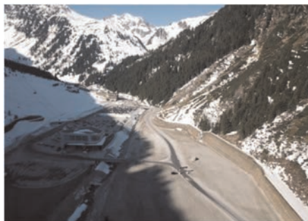
Figure 6. Rockfall protection dam Eisgratbahn-Stubaital.
