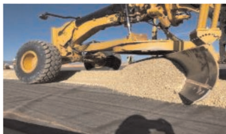
Figure 4b. Equipment and material over BGM.
