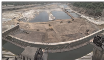
Figure 8. Execution of multistage secondary apron (Kapadia 2020).
