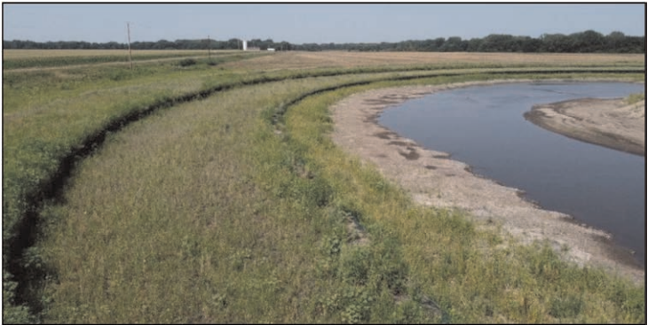
Figure 8. Vegetated SCOURLOK and ARMORMAX performance, July 2021.
