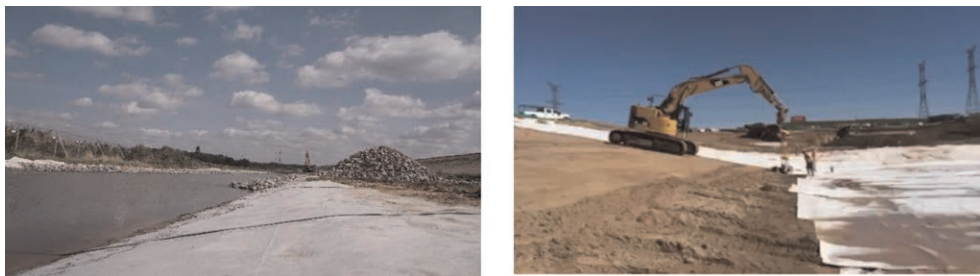
Figure 2. Fully hydrated and/or stubborn groundwater GCL applications in Dyke and/or Canal and/or Pond Applications. Double nonwoven scrim-reinforced GCL being deployed. These GCLs are more robust to installation stresses, have a higher peel than other low grade standard GCLs, and are more weather resistant.
