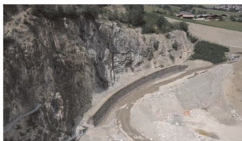
Figure 7. Rockfall protection dam Tenneck.
