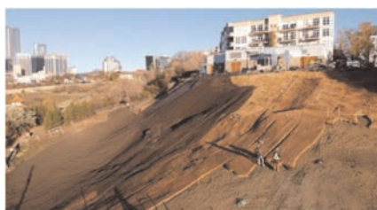
Figure 6. Installation of geocell.
