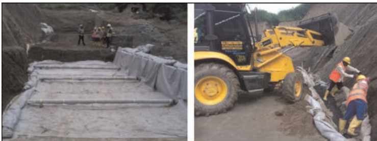
Figure 6. Placement of drainage pipe (left) and drainage blanket at the back of the slope (right).
