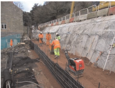
Figure 2. Wall under construction.
