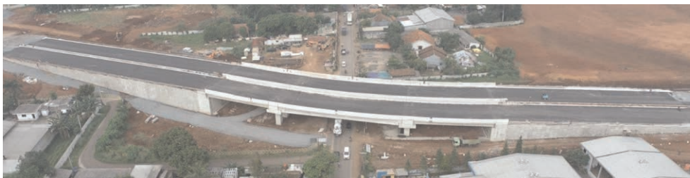
Figure 1. Kadusirung Flyover, Banten, Indonesia.
