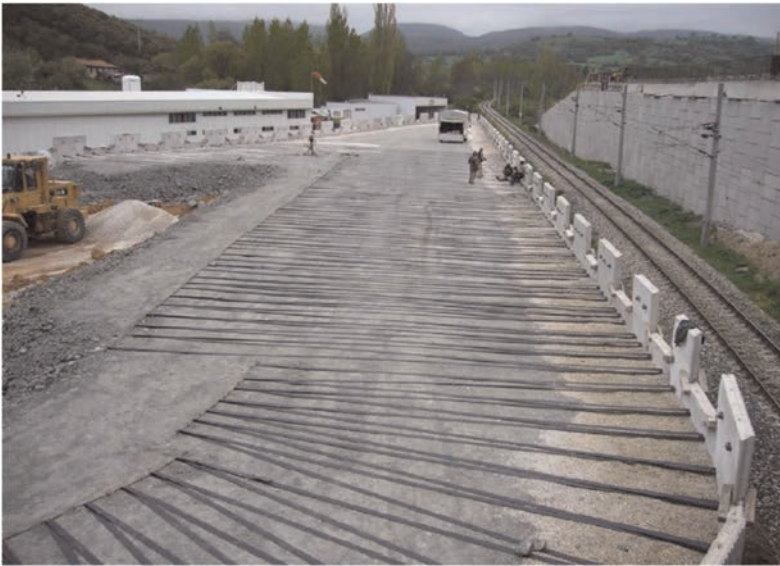
Figure 1. Polymeric strips extending from the rear side of the concrete panel.
