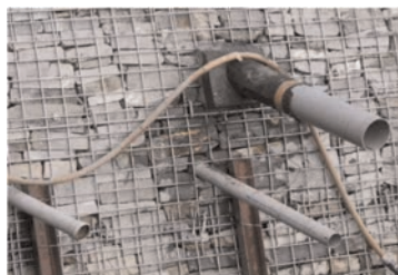
Figure 12. Sub-surface drainage outlets.
