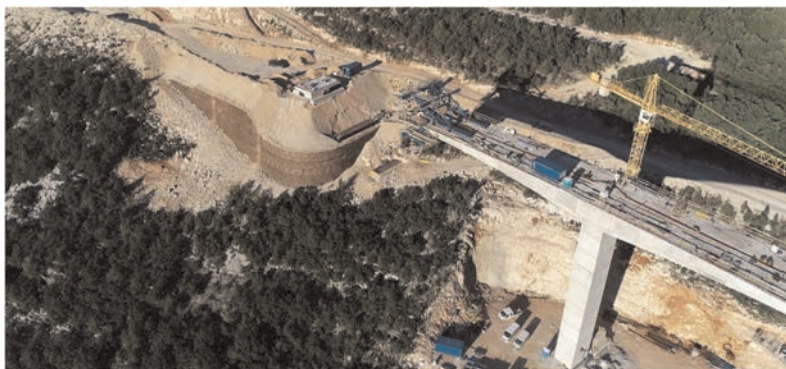
Figure 6. Aerial drone view of the U0 wing wall and abutment of the Dumanja Jaruga viaduct made with the reinforced soil technique with extruded HDPE mono-oriented geogrids.
