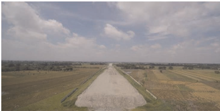
Figure 4. Placement of drainage sand blanket layer prior to placement of geotextile reinforcements.
