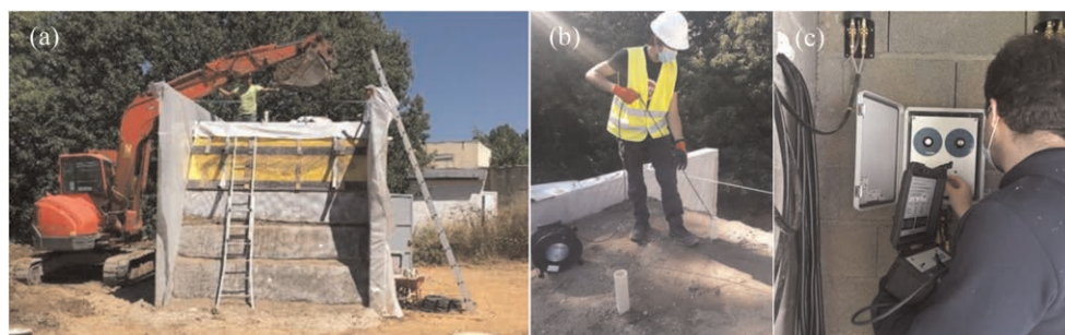
Figure 3. Full-scale instrumented geosynthetic-reinforced structure: (a) during construction; (b) readings on the inclinometers; (c) pressure cells readings.
