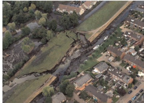
Figure 3. Aerial picture peat levee collapse, caused by dehydration during extreme draught, 2003 Wilnis Netherlands.
