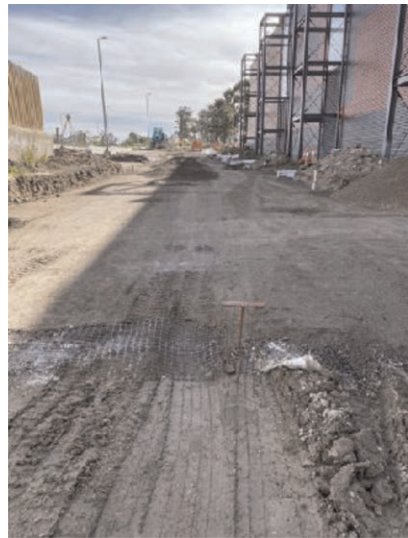
Figure 4. Final pavement ready for asphalt wearing course.
