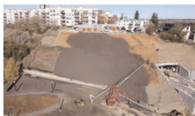
Figure 7. Filling of geocell.
