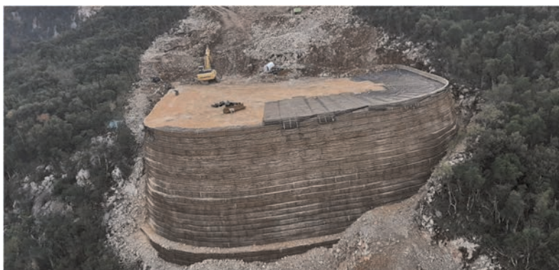
Figure 8. Front drone view of the U4 wing wall and abutment of the Dumanja Jaruga viaduct constructed using a wrap-around reinforced soil technique with a sacrificial steel mesh formwork at the face and mono-oriented extruded geogrids in HDPE.
