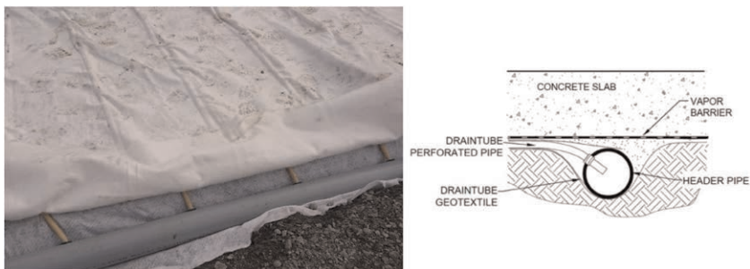
Figure 3. Connection to the header pipe.
