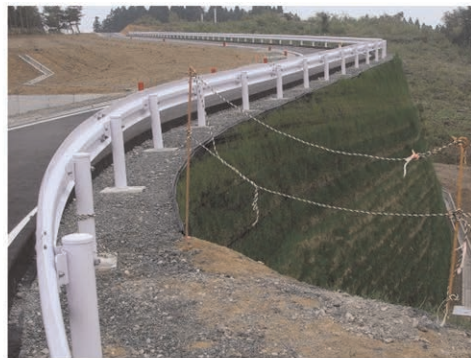
(b) Greened wall facing
