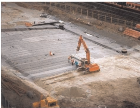
Figure 8a. Membrane installation.
