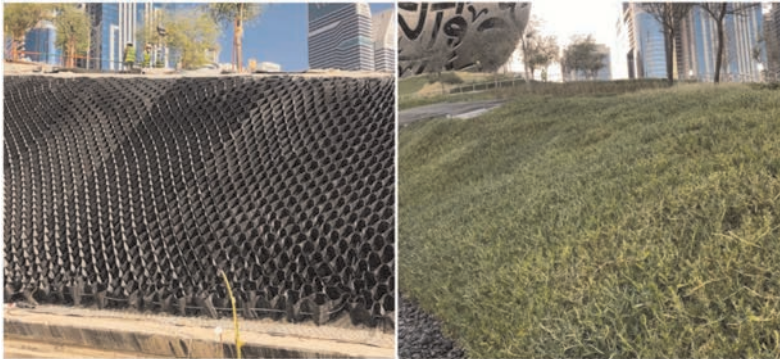
Figure 7. Geocell: before and after vegetation growth.
