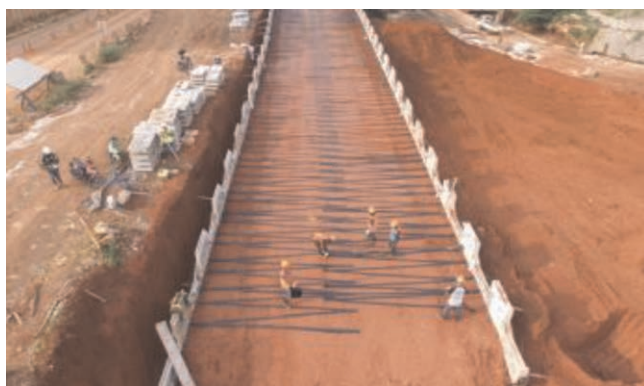
Figure 2. Construction of geoforce segmental retaining wall system.
