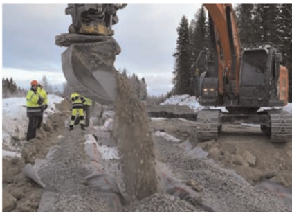
Figure 6. Filling of the trench with granular material.
