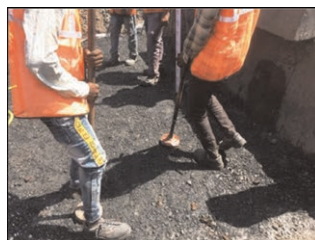
Figure 14. Watering and compaction of infill.
