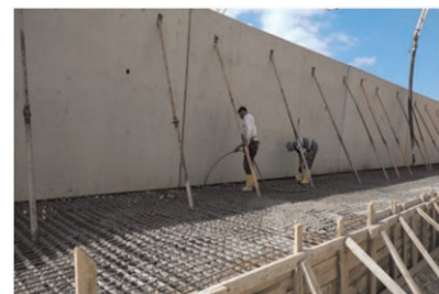
Figure 4d. Pouring of concrete.
