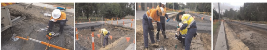
Figure 2. Subgrade preparation and testing.
