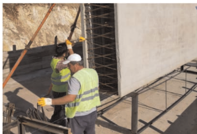
Figure 4c. Installation of horizontal continuity reinforcements.
