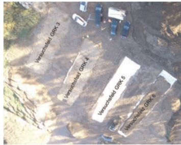
Figure 3. Four test fields at different stages of installation of GTX-NWs.
