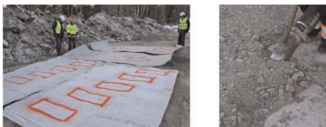
Figure 5. Installed geosynthetic samples with drainage function and recovery of the drainage composites.
