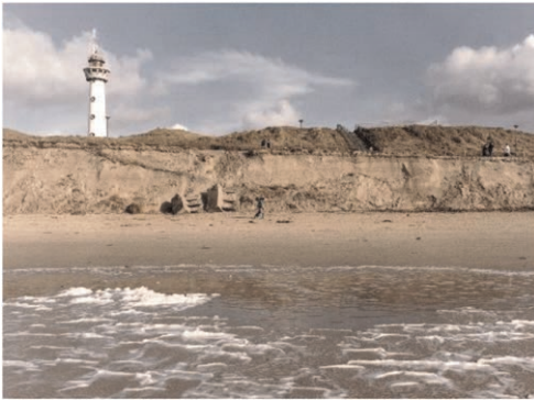
Figure 2. Severe dune erosion after storm surge, Egmond aan Zee lighthouse, The Netherlands.
