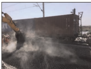
Figure 13. Infilling the geocells.
