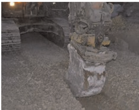
Figure 9. Removal of top part of granular material by excavator.
