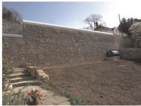
Figure 3. Finished wall with masonry reattached.
