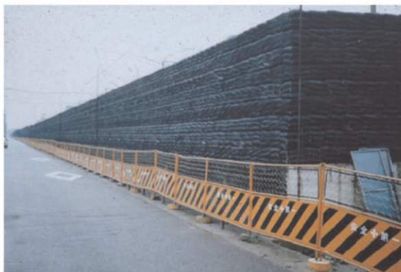
Figure 3. Finished GRS embankment prior to cast-in-situ RC wall construction (Tatsuoka 2018).
