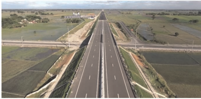
Figure 6. The CLLEx completed with pavement constructed on top of the reinforced embankment.
