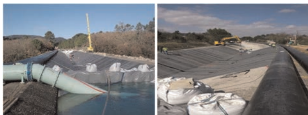
Figure 12. Dewatering work on a section without interrupting water circulation.
