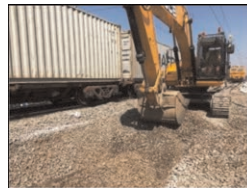
Figure 6. Removal of ballast.
