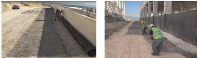
Figure 5. Installation of geogrids.
