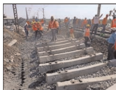
Figure 16. Placing sleepers over ballast.
