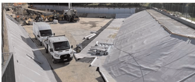
Figure 8. Photo of the geocomposite placing activities.
