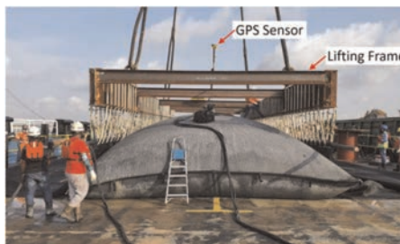
Figure 6. Connecting the lifting frame with geogrid sheet after geotextile tube was fully filled (Geogrid sheet was placed beneath the geotextile tube prior to infilling operation).
