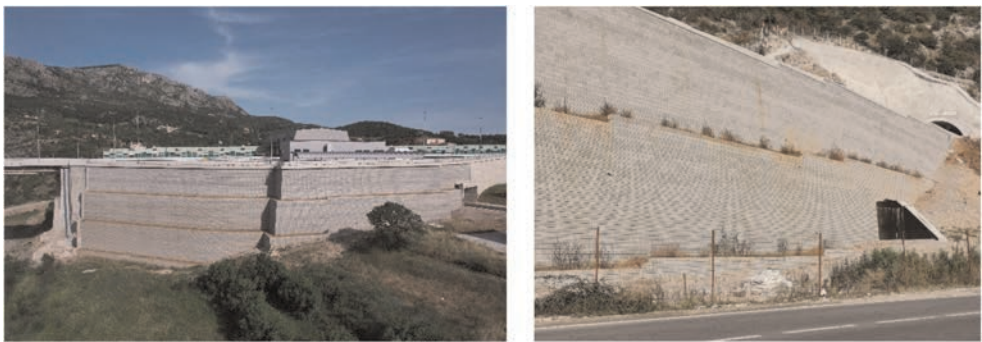
Figure 7. a) Angular wall for highway widening at toll station; b) Wall at tunnel entrance.
