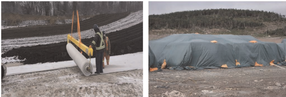
Figure 1. Winter deployment and GCL rolls being stored over the winter until deployment. A GCL made with a dry bentonite can be stored without any concern over the winter season outside until required for deployment.
