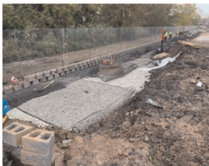
Figure 3. Photo of AASHTO #57 installation.
