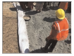
Figure 10. Infilling 100mm thick blanket layer.
