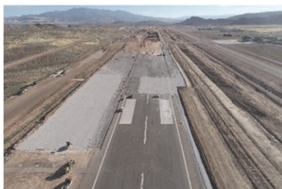
Figure 4a. General view of the site.
