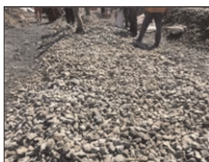
Figure 15. Laying ballast over the blanket layer.
