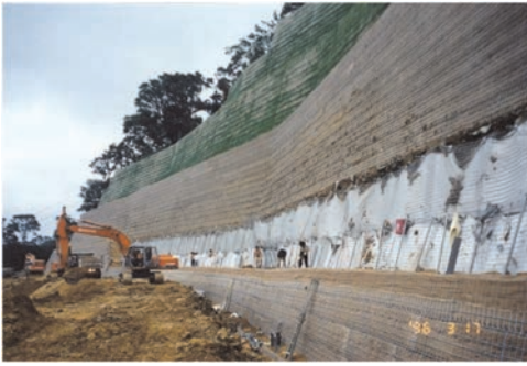
Figure 5. High top-down rock anchored slope with hybrid RSS vegetated slope facing, Taiwan 1996 (AllToffs).
