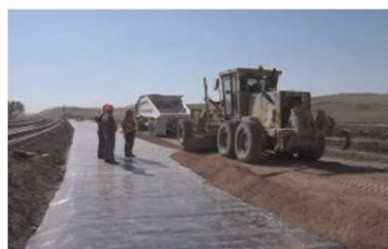
Figure 6b. Sub ballast placement directly on BGM.
