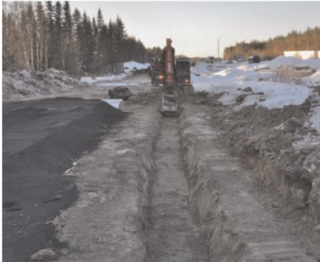
Figure 4. Excavation of trench.
