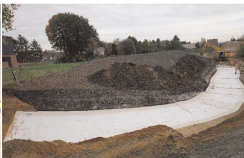
Figure 12. Horizontal installed Geosynthetic Clay Liner (GCL) in the levee foreland to enlarge the seepage length from the flood defense base.
