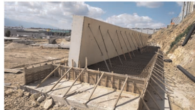
Figure 4b. Formwork of foundation and installation of steel reinforcement.
