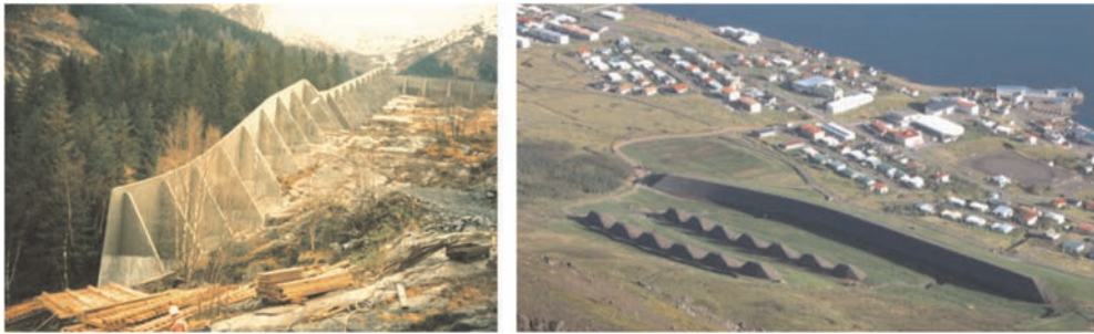
Figure 1. Examples of reinforced concrete (RC) wall (left) and MSE walls (right) used as protection structures (Barbolini et al. 2009).
