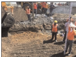
Figure 8. Checking the excavation level.
