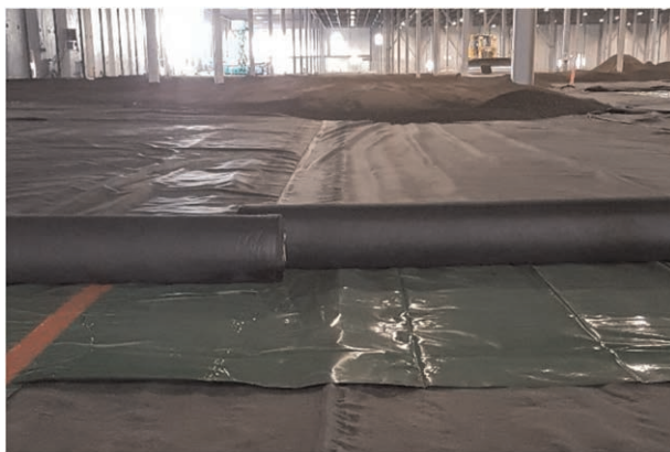
Figure 4. Vapor barrier and geotextile installation.
