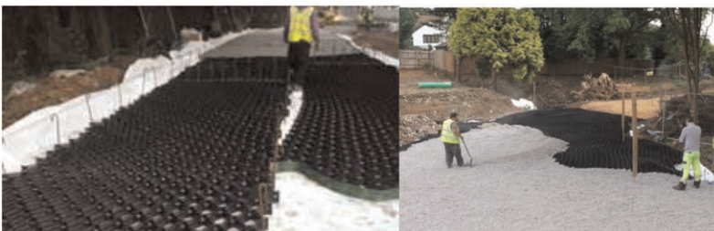
Figure 3. Cellweb system with clean angular stone & geotextile for separation beneath it.
