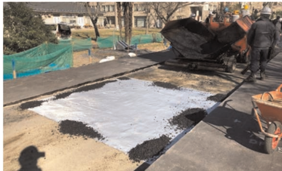
Figure 3. Placement of geotextile PET at 200 mm from the surface of prototype scale model test road.
