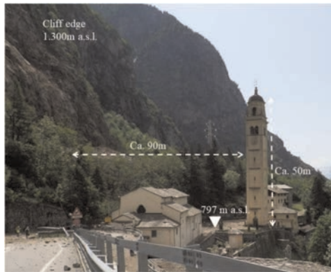
Figure 1. View of the Sanctuary area from national road 36.
