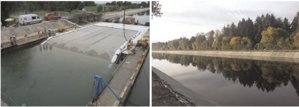
Figure 5. Canal sealing: during installation from pontoon (left); after installation (right).
