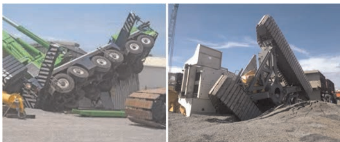
Figure 1. Examples of construction machinery overturning.
