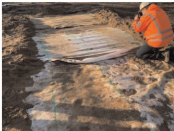
Figure 6. Stretched sample and relaxed sample after removal of fill material.
