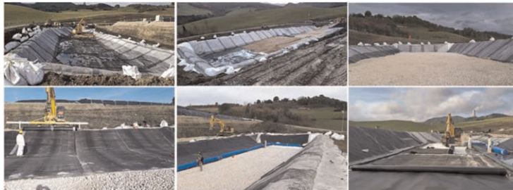
Figure 2. Installation phases of the base reclamation (left to right): 1. Nonwoven and geogrid, 2-3. Aggregate layer, 4-5. Rough bentonite geocomposite, 6. Rough HDPE geomembrane.
