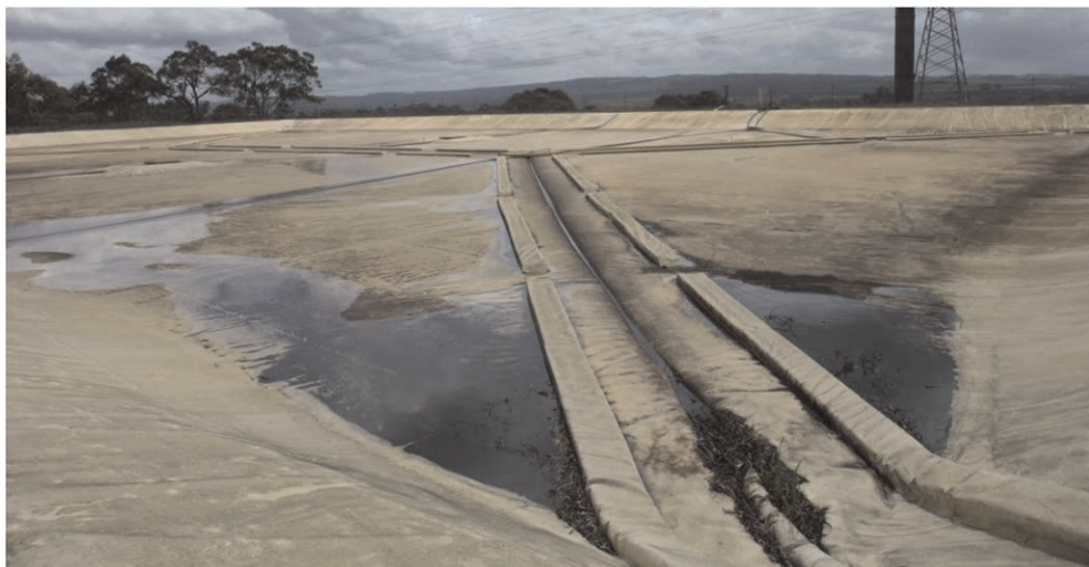
Figure 6. A floating cover with foam floats for tensioning and other floats for access walkways.
