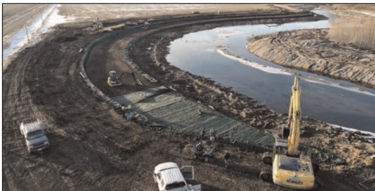
Figure 7. Installation of SCOURLOK and ARMORMAX, January 2021.
