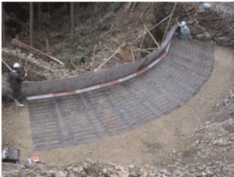
(a) During construction
