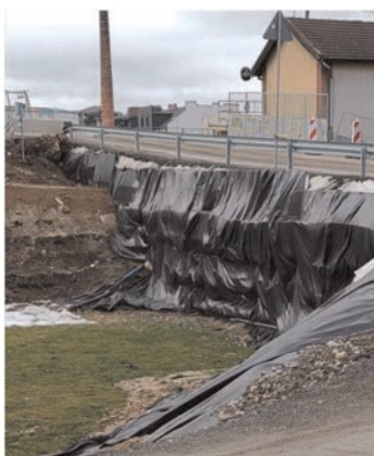
Figure 8. Bypass temporary construction – facing.
