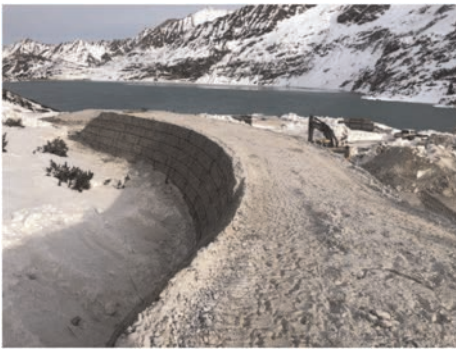
Figure 2. Tauernmoos avalanche deflecting dam during construction. (Nov. 2021).
