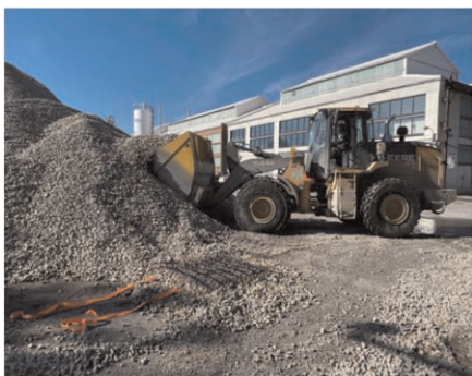
Figure 1. Photograph of UL-FGA installation.
