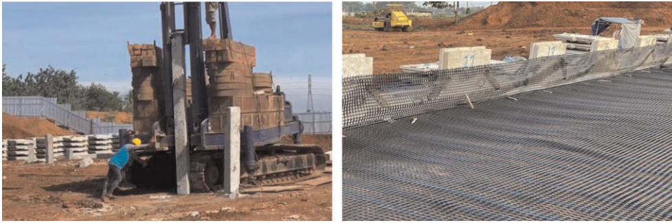
Figure 3. Geosynthetics reinforcement scheme in piled embankment system.
