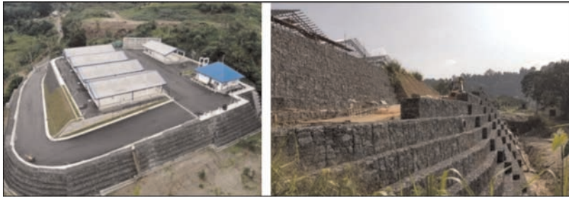
Figure 7. Completion of reinforced soil retaining slope.
