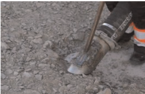
Figure 4. Removing soil with the vacuum / sucking lorry.
