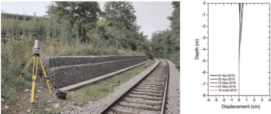
Figure 4. Retaining structure after completion (left) and horizontal displacements in borehole above the retaining wall (right).
