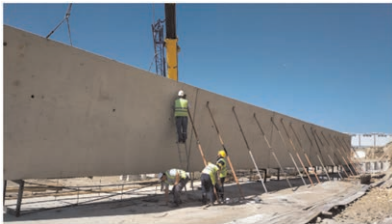
Figure 4a. Installation and propping of double wall modules.
