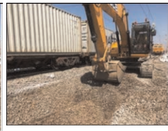
Figure 7. Removal of sub-ballast/blanket.
