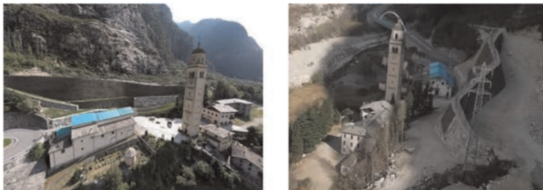
Figure 6. Aerial views of the finished works.
