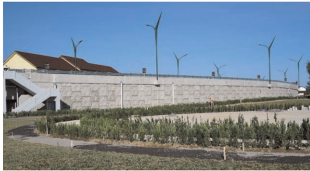
Figure 1. Kretek II Flyover's, Yogyakarta, Indonesia.
