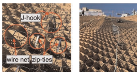
Figure 5. Installation of wire net with geocell.
