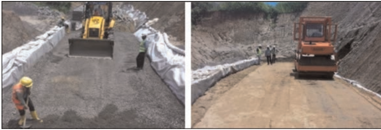
Figure 5. Placement of backfill soil (left) and compaction of backfill soil (right).
