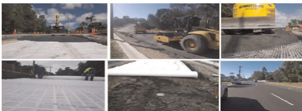
Figure 3. Installation of pressure cell, geocomposite, geogrid, gravel and asphalt.
