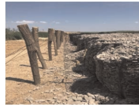
Figure 6. Geomattress filled with a stone material.
