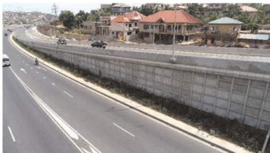
Figure 2. Precast concrete wall panels with artistic 3-D signs.
