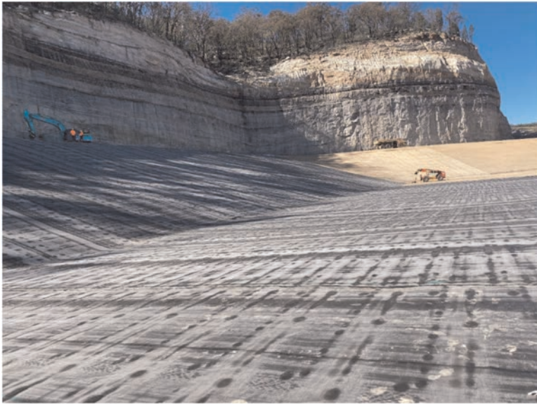
Figure 3. BGM being used for environmental protection by containing stormwater run off from a mine before it reaches the river. New South Wales, Australia.
