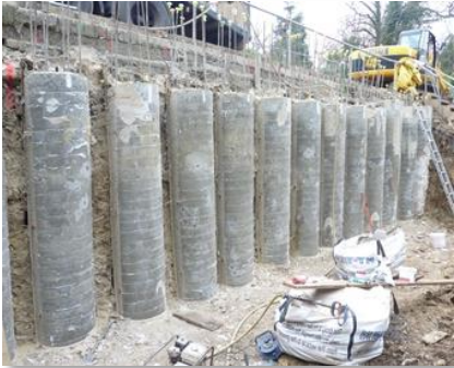
Tangent Pile Walls
