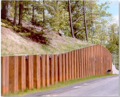
Sheet Pile Walls
