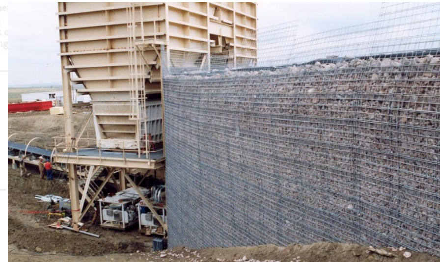
Reinforcement over areas prone to subsidence
