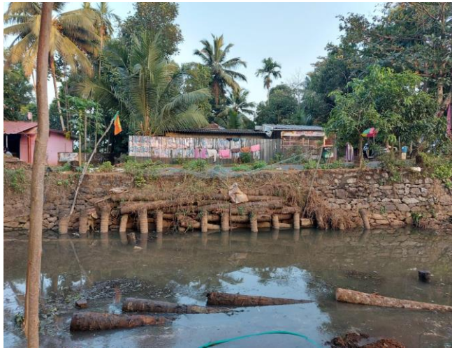
Coconut logs used as piles below bridge abutment in soft clays, Kerala PWD, India
