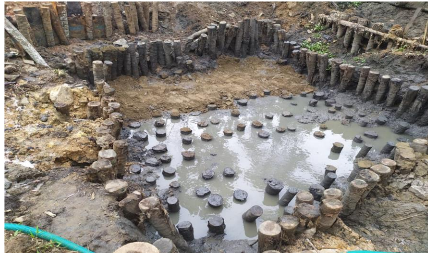
Coconut logs used as piles below bridge abutment in soft clays, Kerala PWD, India
