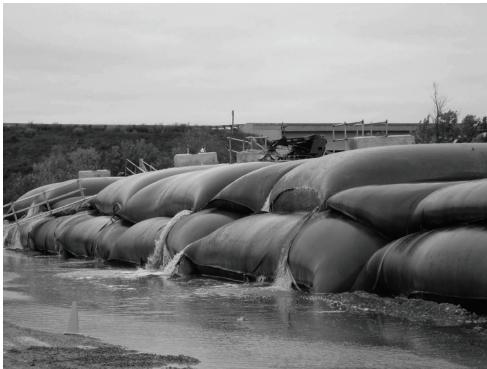
b) Sediment dewatering within geotextile tubes
