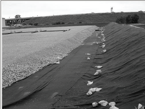
a) Lined drainage blanket beneath geotextile tubes
