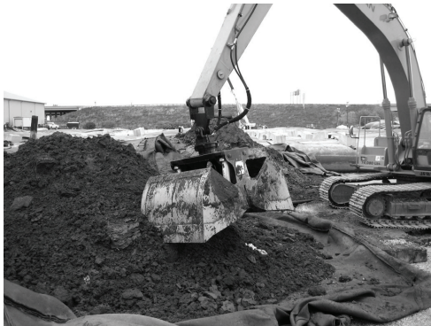
c) Removal of dewatered sediment from geotextile tubes
