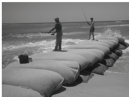
c) Geotextile bags
