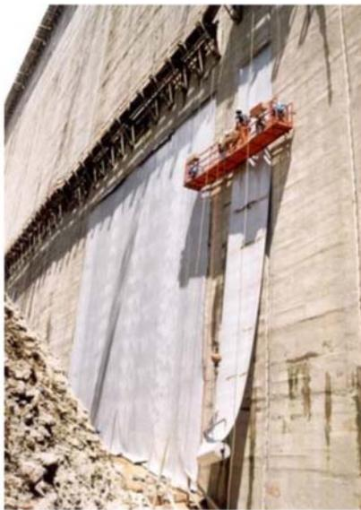
Lining the upstream face of a dam<sup>(\*)</sup>
