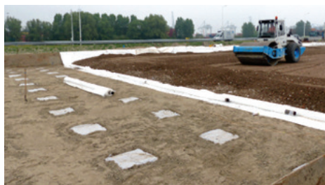
Reinforcement over piles with high strength wovens
