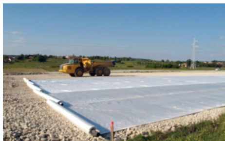
Permanent reinforcement for railways embankment
