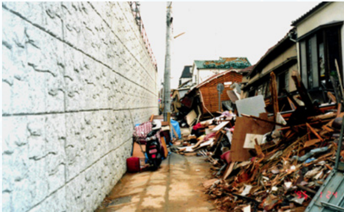
Fig.2 Surveyed reinforced wall during the Kobe earthquake (Tatsuoka et al: S&F, 1996)
