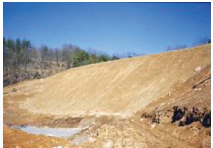
Completed reinforced embankment
