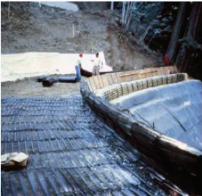
Example remediated slope with reinforced slope structure
