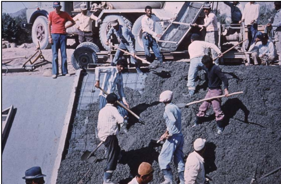
Placing concrete on slopes was labor-intensive. Archive J.P. Giroud
