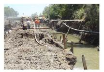
Figure 1Diversion channel running parallel to canal lining works
