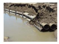
Figure 2: Canal diversion on IIIMP in Egypt while constructing a U-Section concrete lining
