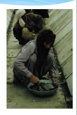
FESS Project Pakistan: Placing precast slabs on bed and precast side panels
