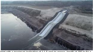
Inlet with a maximum inclination of 1:1,5 and an approx. length of 160 m for a
