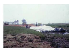
Construction of a reinforced unpaved road on soft organic clay
