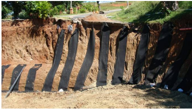
Figure 3. Wall Drainage Systems
