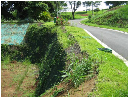
Figure 10. Vegetative state of the facade two months after construction
