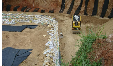
Figure 6. Compaction of the soil: density greater than 95% of Modified Proctor
