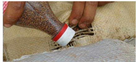
Figure 8. Vegetation seeds installed in each sack
