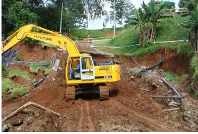
Figure 2. Preparation of the site for the construction of the wall
