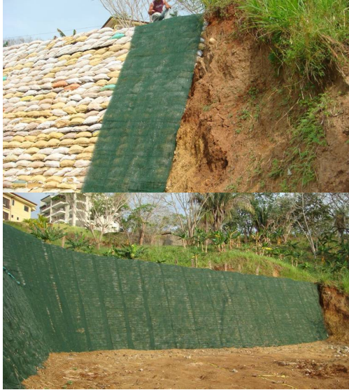
Figure 9. Installation of the permanent erosion control mat: TRM435
