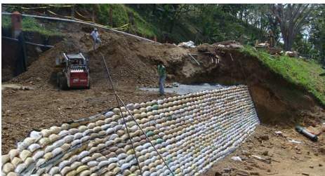
Figure 5. Installation of the woven geotextile and spread of the fill soil
