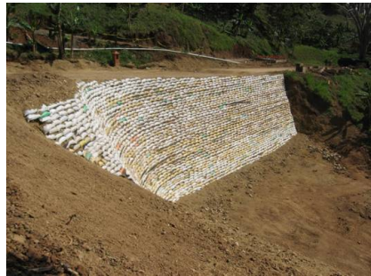
Figure 7. Facade of the wall with sacks filled with organic soil
