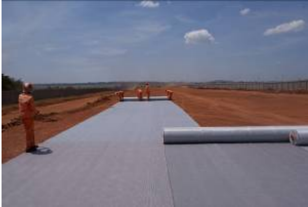
Figure 61: Geogrid reinforced foundation for Gautrain rapid rail route over dolomitic area
