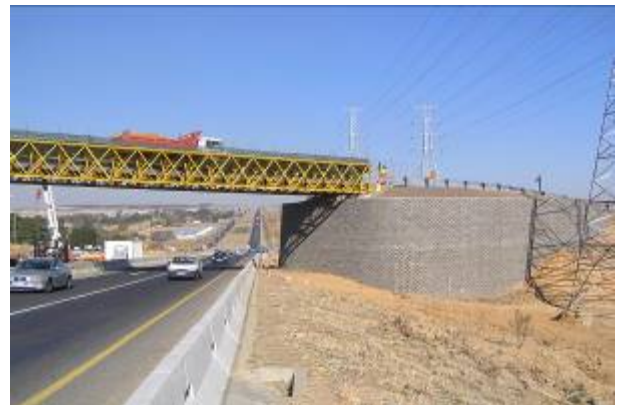
Figure 64: Geogrid reinforced soil abutment for construction vehicle overpass on Gautrain route
