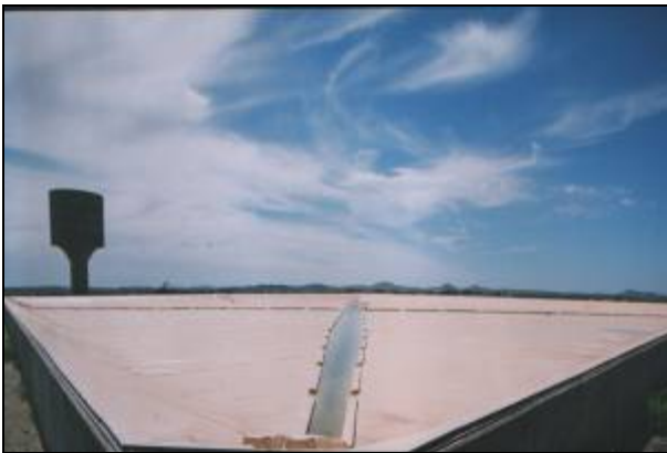
Figure 17: Floating cover and membrane lined potable reservoir in Africa
