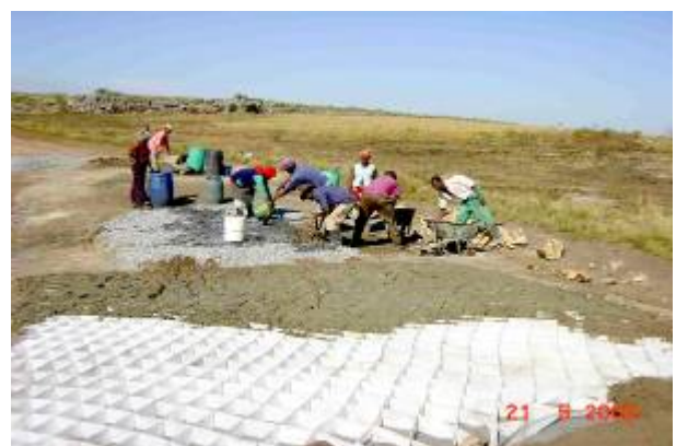
Figure 68: Geocell drift construction on Amadiba Road poverty alleviation project
