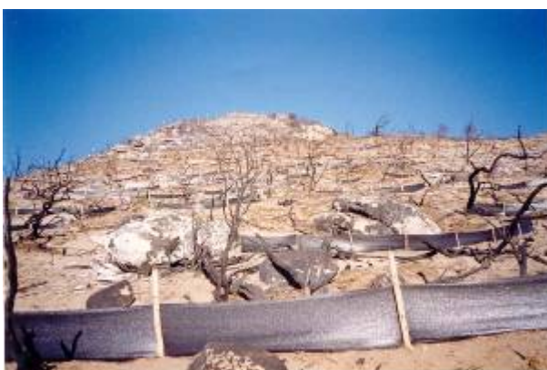
Figure 67: Silt fence after vegetation destruction by fire
