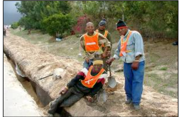
Figure 70: Mole Rat barrier installation
