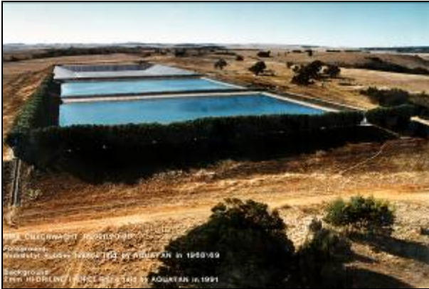
Figure 15: Onverwacht raw water reservoirs: HDPE lined earth embankment reservoir and refurbished concrete reservoir lined with HDPE
