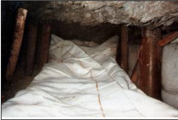
Figure 55: Backfill bag support in deep level gold mining
