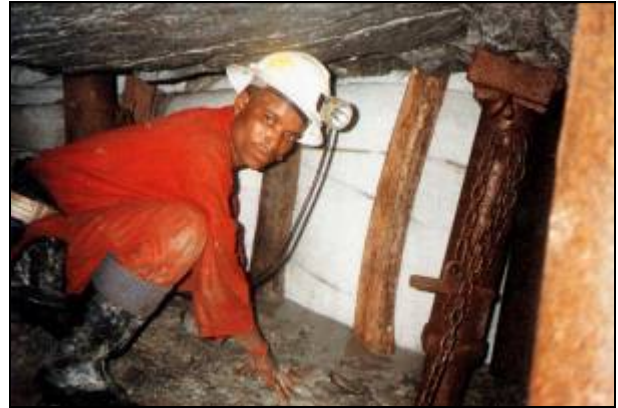
Figure 56: Backfill bag support in deep level gold mining
