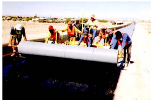
Figure 66: Paving fabric in road rehabilitation, Namibia
