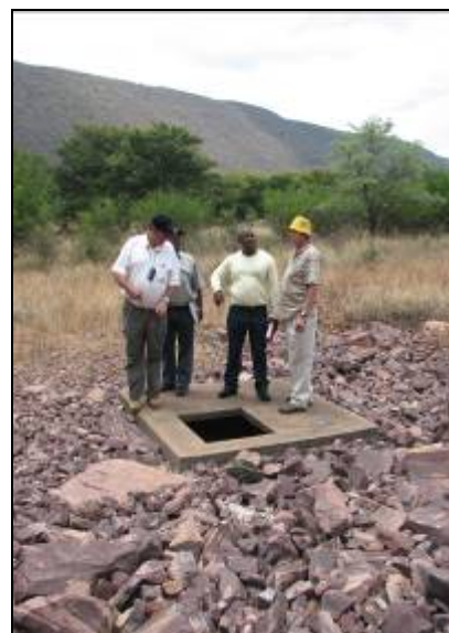
Figure 4: Seepage monitoring well
