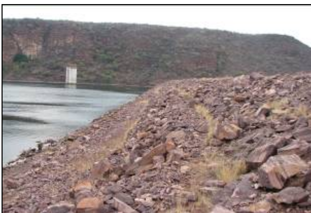
Figure 3: Completed dam as at 2008
