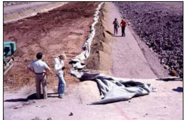
Figure 2: Geotextile adjunct between core and graded filters
