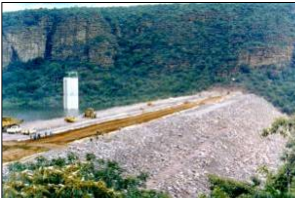
Figure 1: Embankment under construction
