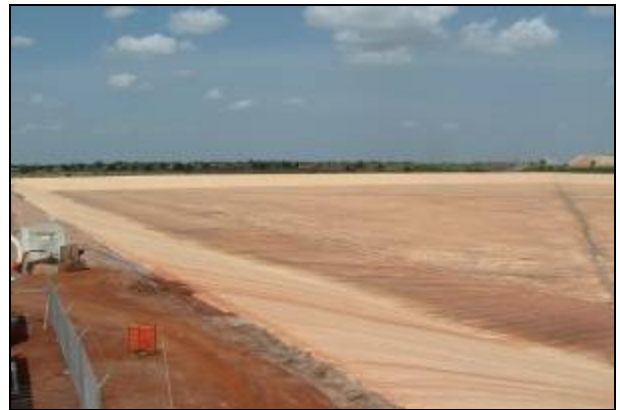
Figure 18: Floating cover and membrane lined potable reservoir in Africa
