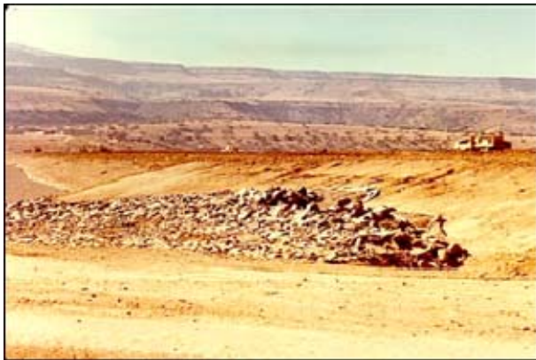
Figure 7: Geotextile under riprap on upstream face
