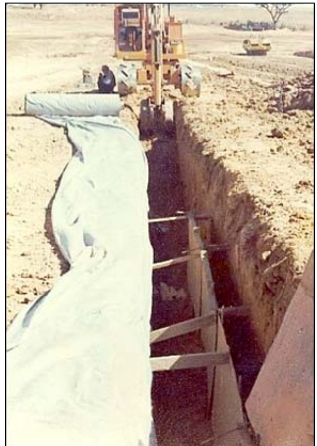
Figure 8: Internal filter downstream interface of chimney drain
