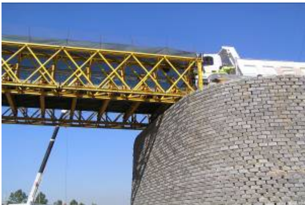
Figure 63: Geogrid reinforced soil abutment for construction vehicle overpass on Gautrain route
