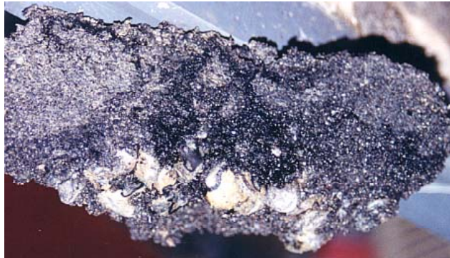
Figure 4. The sand layer of the granular filter system experience significant clogging. Concreted zones of cemented sand and pea gravel created a zone of reduced permeability and perched leachate mounding within the waste once the sand layer clogged. Reproduced from Mclsaac, R. and Rowe, R.K. (2006) Effect of filter/separators on the clogging of leachate collection Systems, Canadian Geotechnical Journal , 43 (7): 674-693 with permission of the Canadian Geotechnical Journal.
