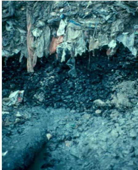
Figure 1. Partial clogging of the unsaturated and saturated coarse (50mm) gravel layer after 4-5 years as reported by Fleming et al. (1999). This system was still controlling leachate heads to below the design value.
