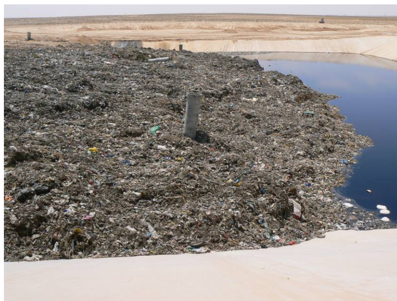
Figure 2. Leachate generated by biodegradation of organic waste at a MSW landfill located in a desert.
