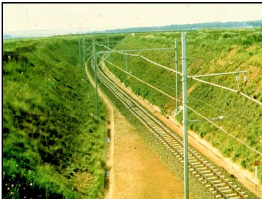
Picture 11 - Completed rail construction
