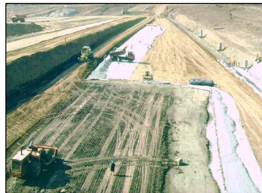
Picture 8 - Geotextile in blanket & toe drains
