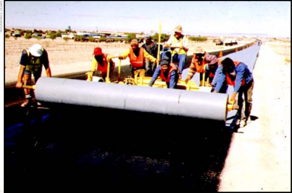
Picture 20 - Paving fabric on road rehabilitation
