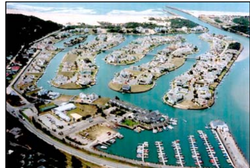
Picture 16 - Construction completed
