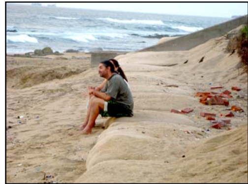
Picture 18 - Repair with geocontainers
