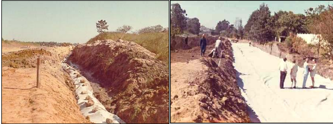
Picture 3 - Subsoil drain in Richards Bay 1973
