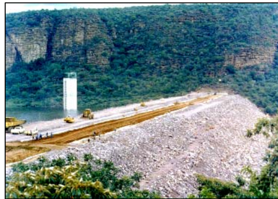
Picture 6 - Geotextile in Mokol Rockfill Dam
