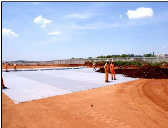
Picture 21 - Geogrid reinforcement
