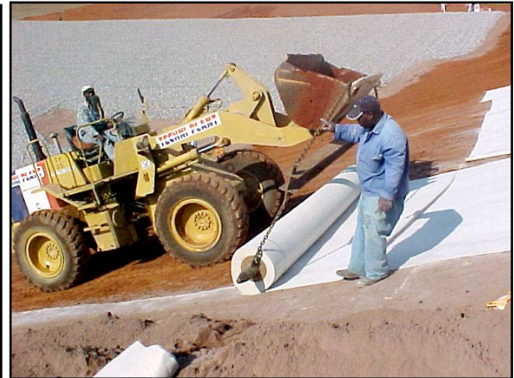
Picture 22 - Geosynthetic Clay Liner (GCL)
