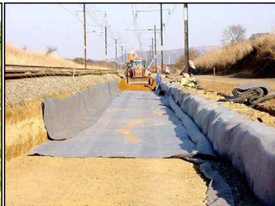
Picture 12 - Special “Coal Line” construction
