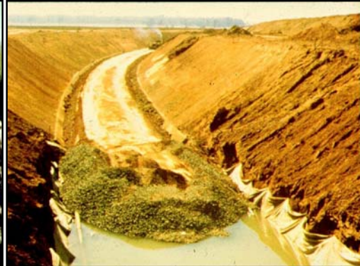
Picture 10 - Geotextile – drainage gravel - formation
