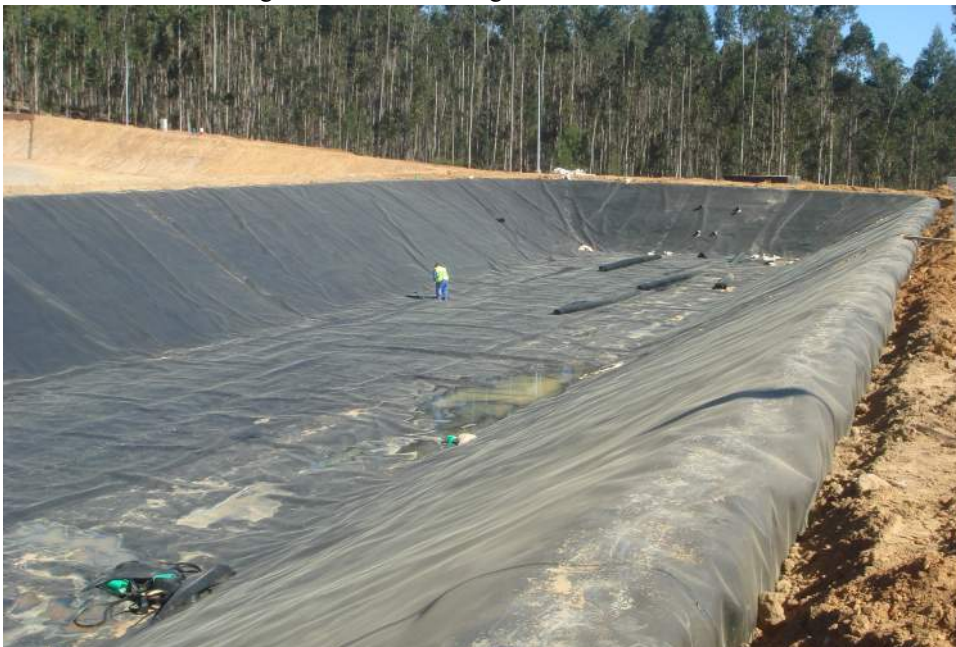
Figure 13. Example of a landfill pond in construction
