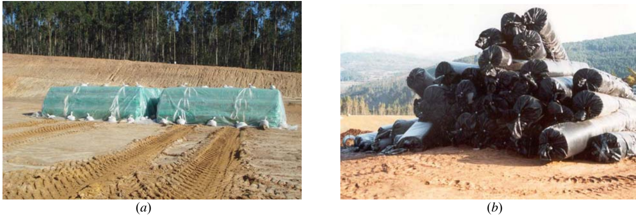
Figure 40. Photographs illustrating (a) good and (b) bad storage of geosynthetic rolls
