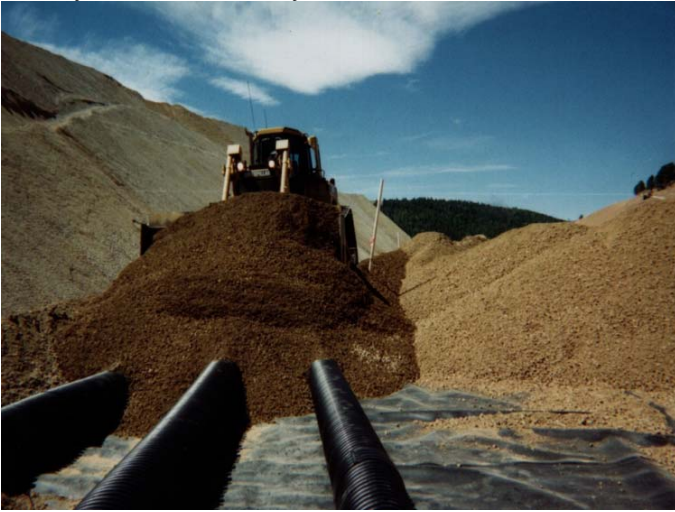
Figure 16. HLP CPe solution collection pipes
