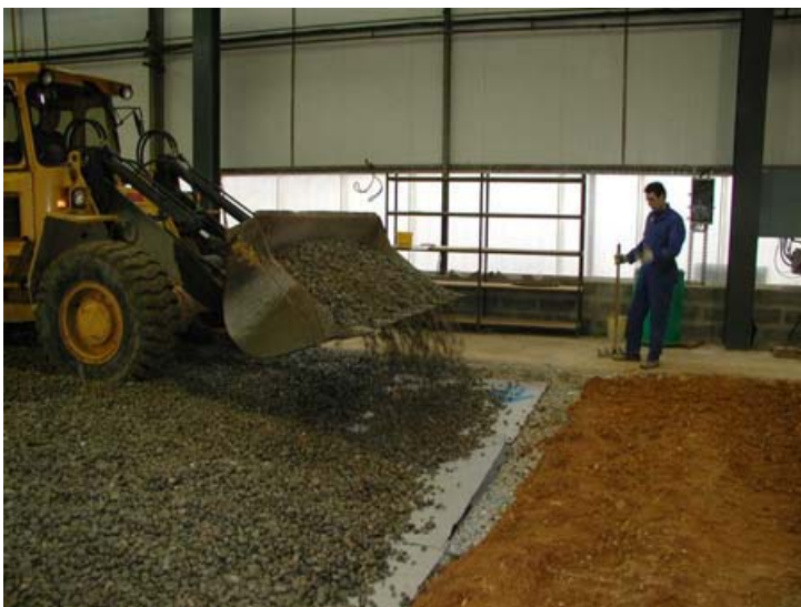
Figure 34. Installation of testing pads (from Khay et al. 2006)
