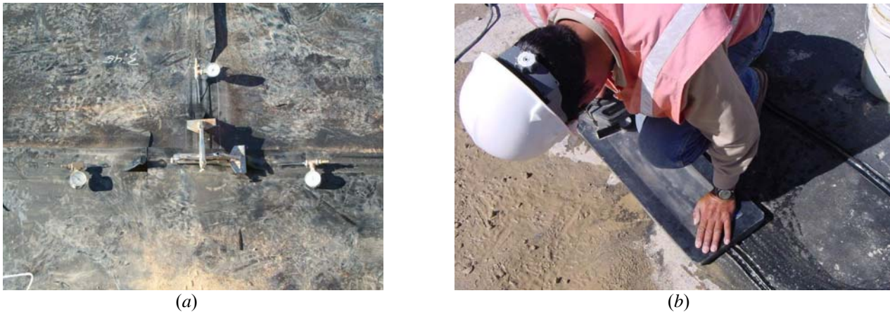
Figure 45. (a) Air Pressure Testing Double Fusion Weld; and (b) vacuum box
