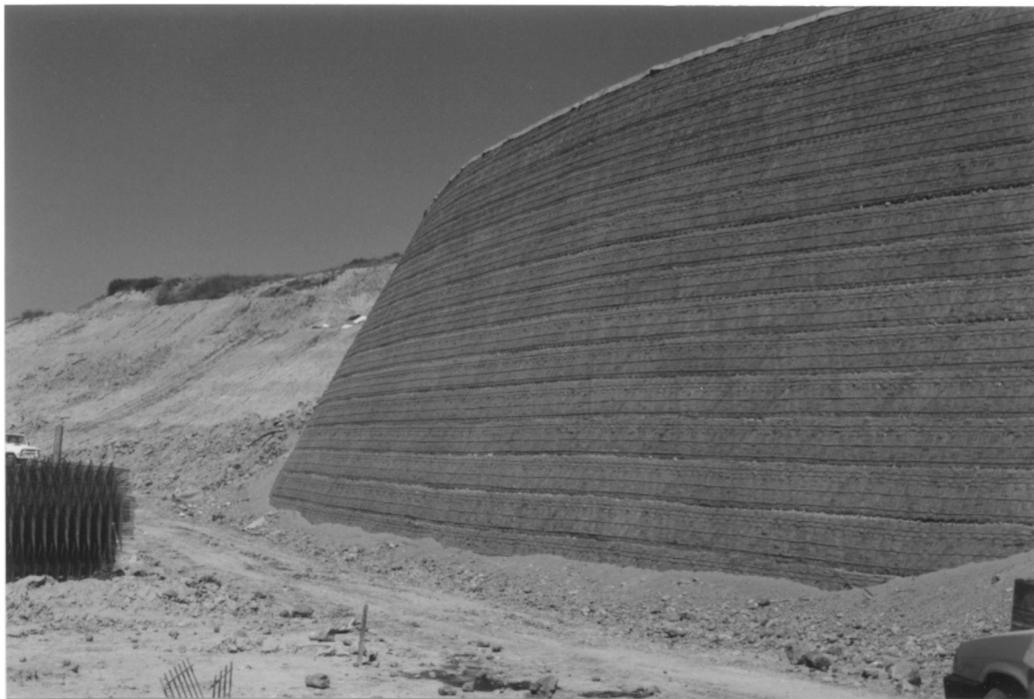
Figure 5. View of the lower wall.
