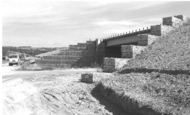
Figure 4. Reinforced gabion walls as highway bridge wings
