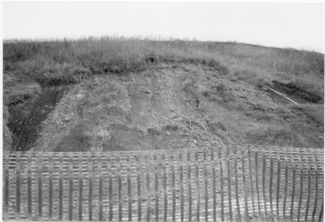
Figure 1. Plate sliding on the landfill slope
