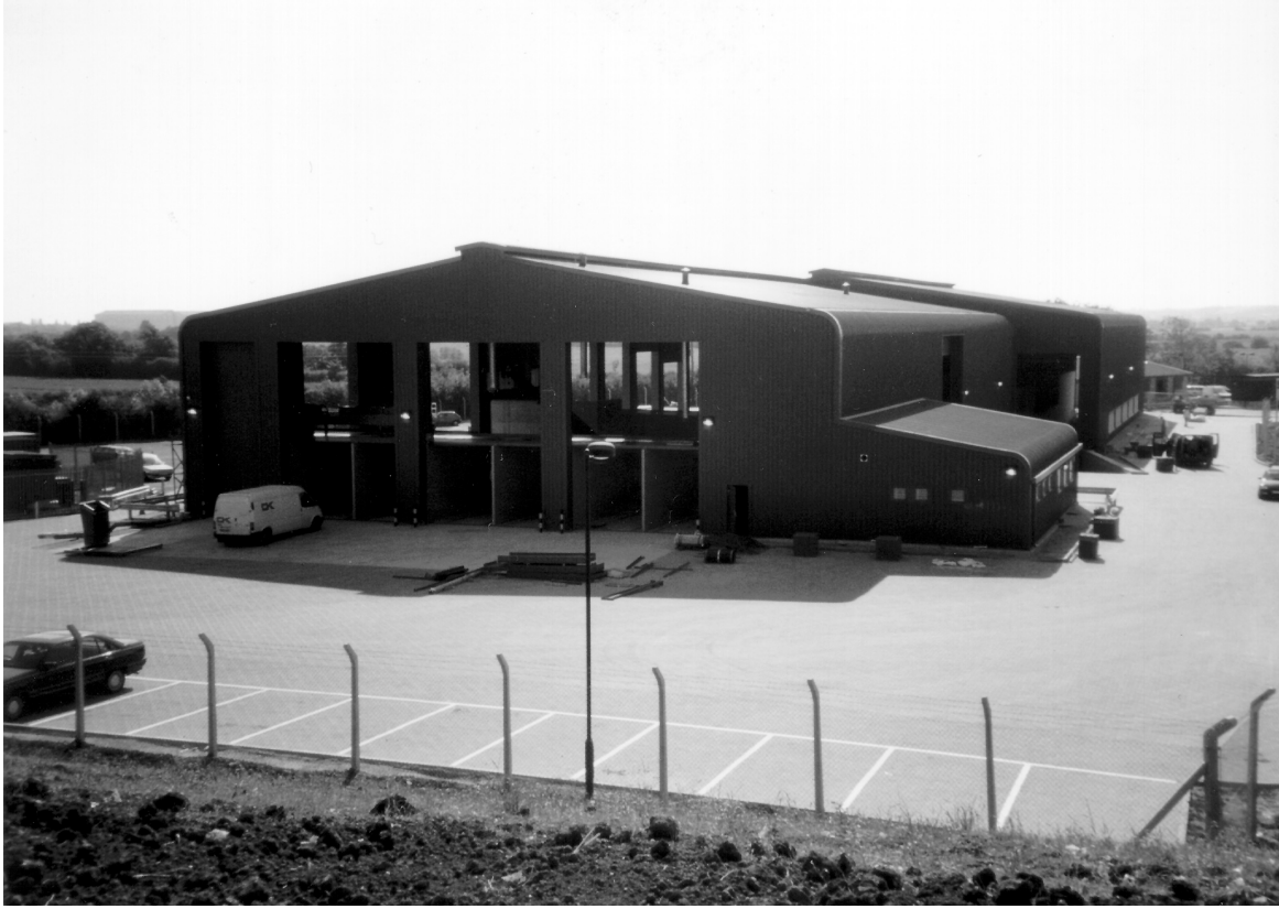
Figure 2. Photograph of the north-west end of Waste Transfer building
