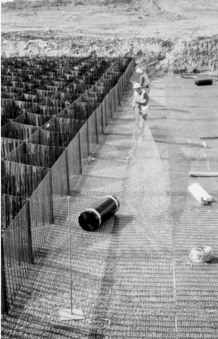
Figure 5. Geocell raft during construction
