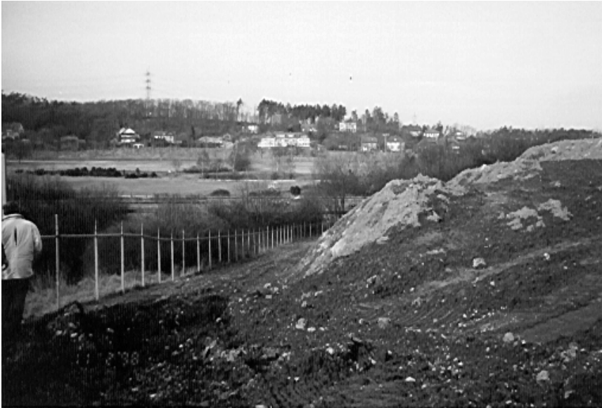
Figure 5: Surface of the construction site in original condition
