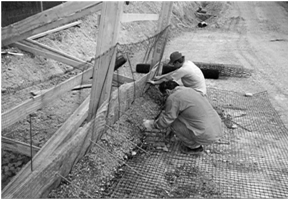
Figure 7: Installation of a wedge of topsoil
