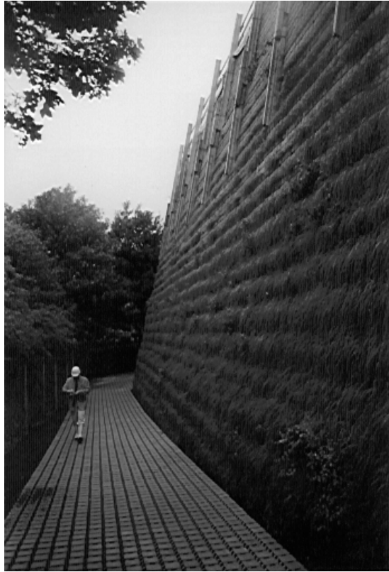
Figure 8: West surface during construction, half complete
