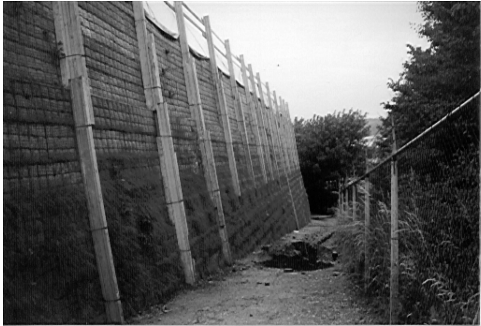
Figure 6: North side of the construction during building
