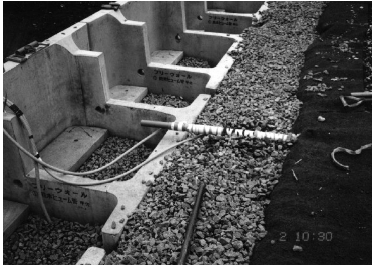
Photo-7 Inclinometer (installation of pipe gage)
