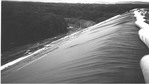
Photo 1. View of the lined slopes before laying of the reinforced geocomposite.
