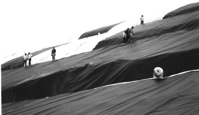
Photo 2. Berms laid by geomembrane and reinforced geocomposite.
