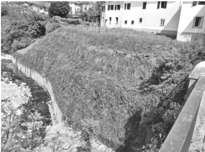
Figure 8. A recent view of the reinforced earthfill (March, 2000)
