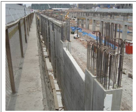
Figure 1: The perimetric retaining walls of the bus station.
