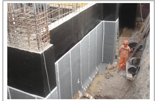
Figure 5: The drainage's geocomposite in the wall.
