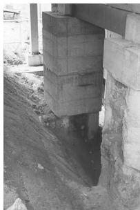
Fig. 1: Situation between the piles
