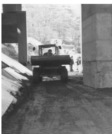
Fig. 3: Soil transport between the piles
