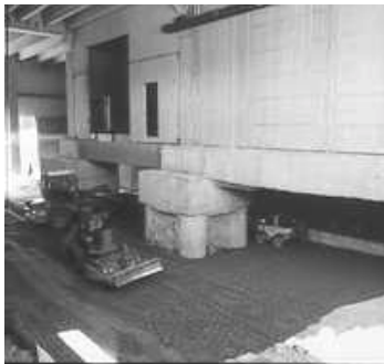
Fig.10: General view of the construction site
