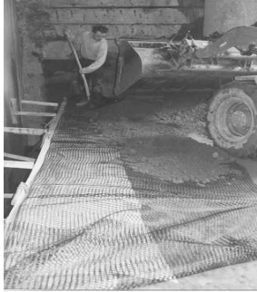
Fig. 8: Installation by hand
