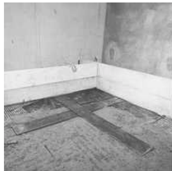
Fig 7: Edge corner of the geosynthetic wall
