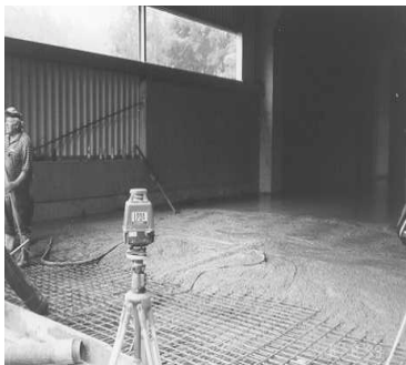
Fig.11: Concrete plate on the second level above the geogrid reinforced wall
