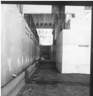
Fig. 6: Geogrid installation between the piles
