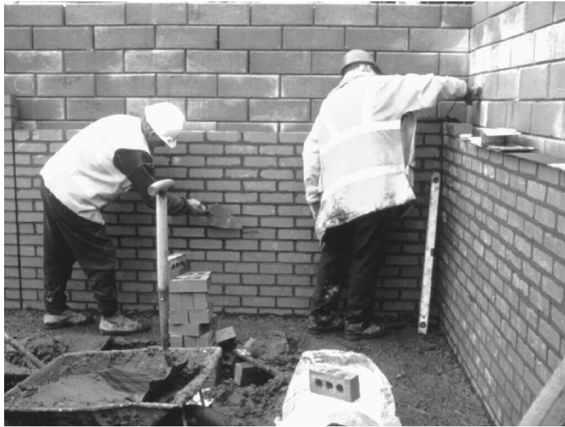
Figure 16. A brick fascia is often chosen to face up the structure
