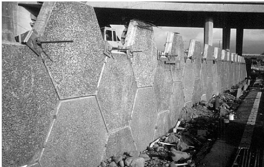
Figure 2. Incremental panel wall
