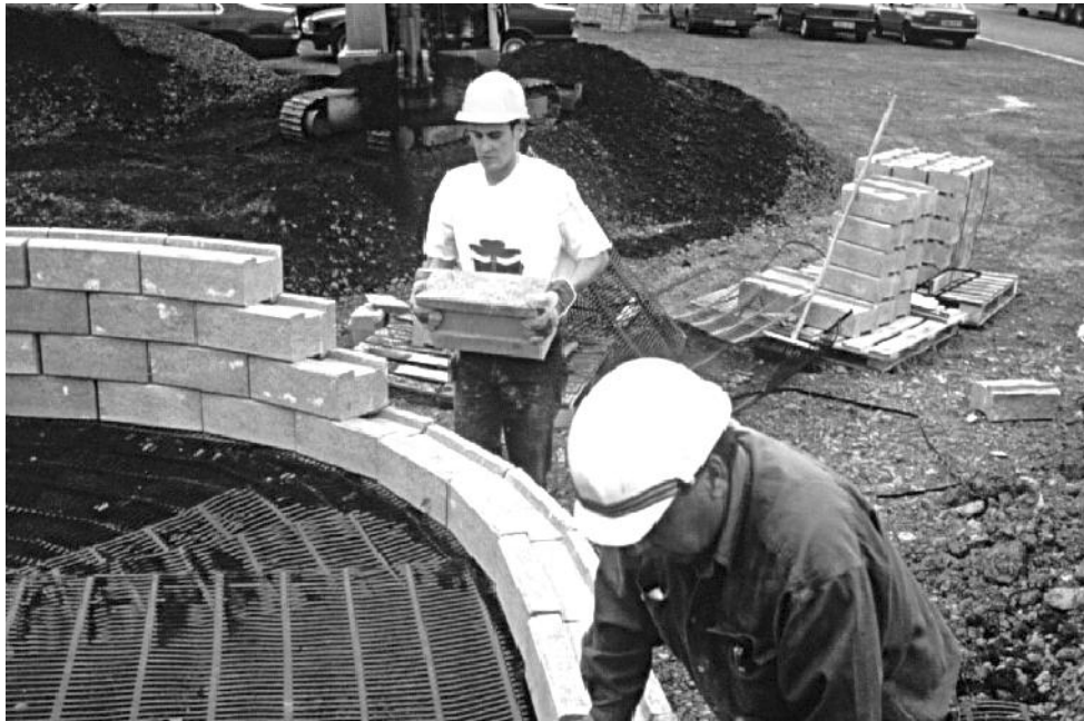
Figure 12. Construction of a horizontal curve
