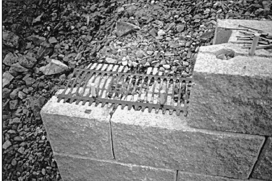
Figure 5. Geogrid connected to face locked together by the use of fibreglass location pins and drainage medium.
