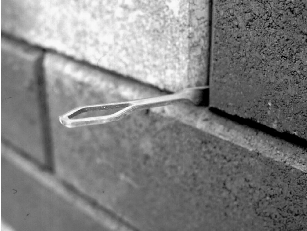
Figure 15 Stainless steel tie fitted into facing unit
