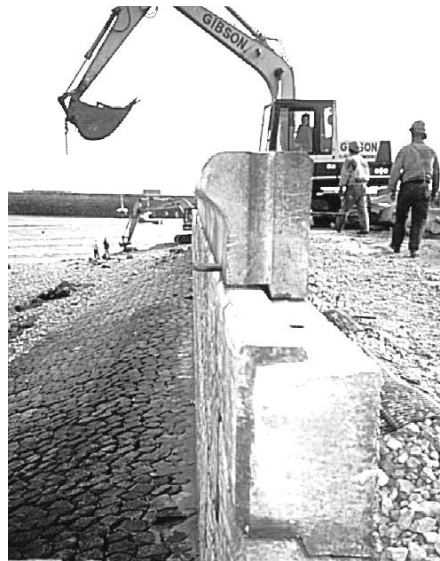
Figure 3. Large incremental unit using cast-in geogrid
