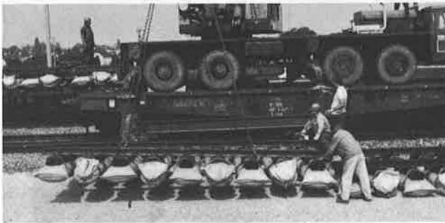
Fig. 9 Placing the elements on the prepared subsoil
