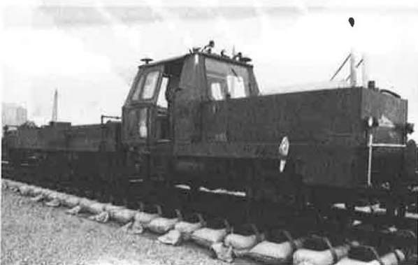
Fig. 10 Preloading by track stabilizer
