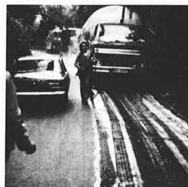
Trial Site 84/2 Applying Chippings
