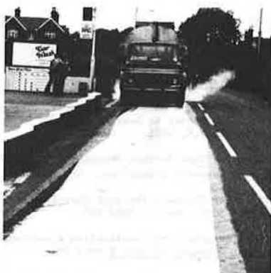
Trial Site 84/2 Rolling out the Fabric
