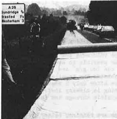
Trial Site 84/1 Rolling out the Fabric
