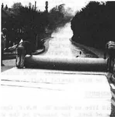
Trial Site 84/2 Rolling out the Fabric
