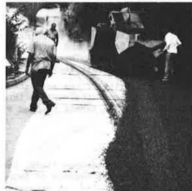
Trial Site 84/2 Applying Chippings
