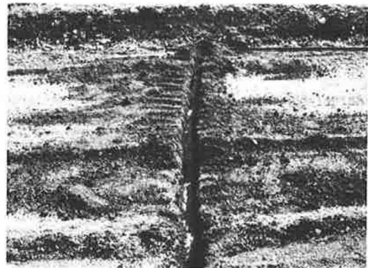
Fig. 12 : Trench in the experimental road
