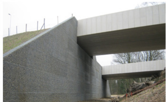
Figure 6. Measurement data of horizontal and vertical deformations during preloading and bridge deck installation as well as pictures of the preloaded retaining wall and finished abutment with installed bridge deck (van Duijnen et al. [2])
