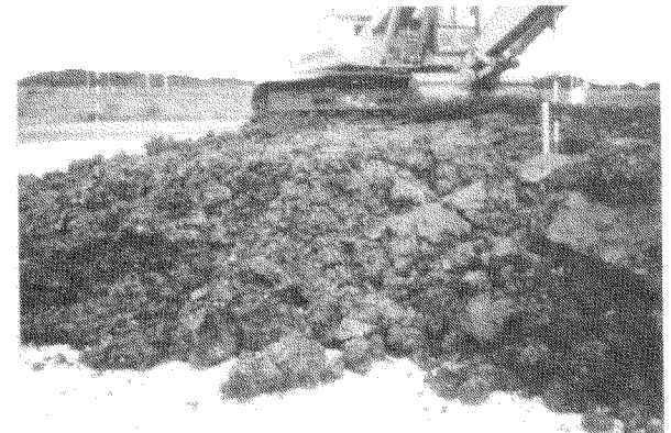
Photo. 2 Banking Material after Excavation and Removal
