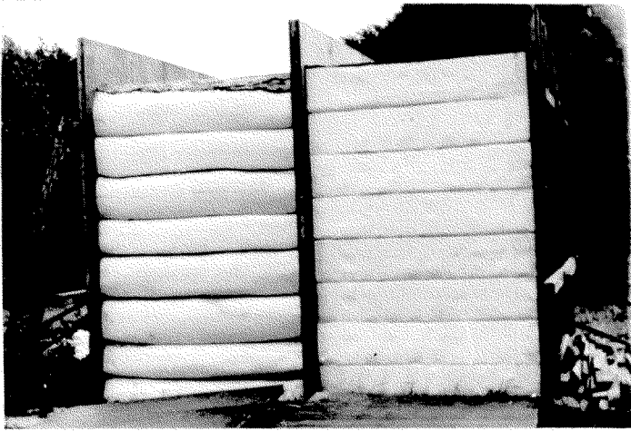
Figure 8 General view of Section 1 and Section 2
