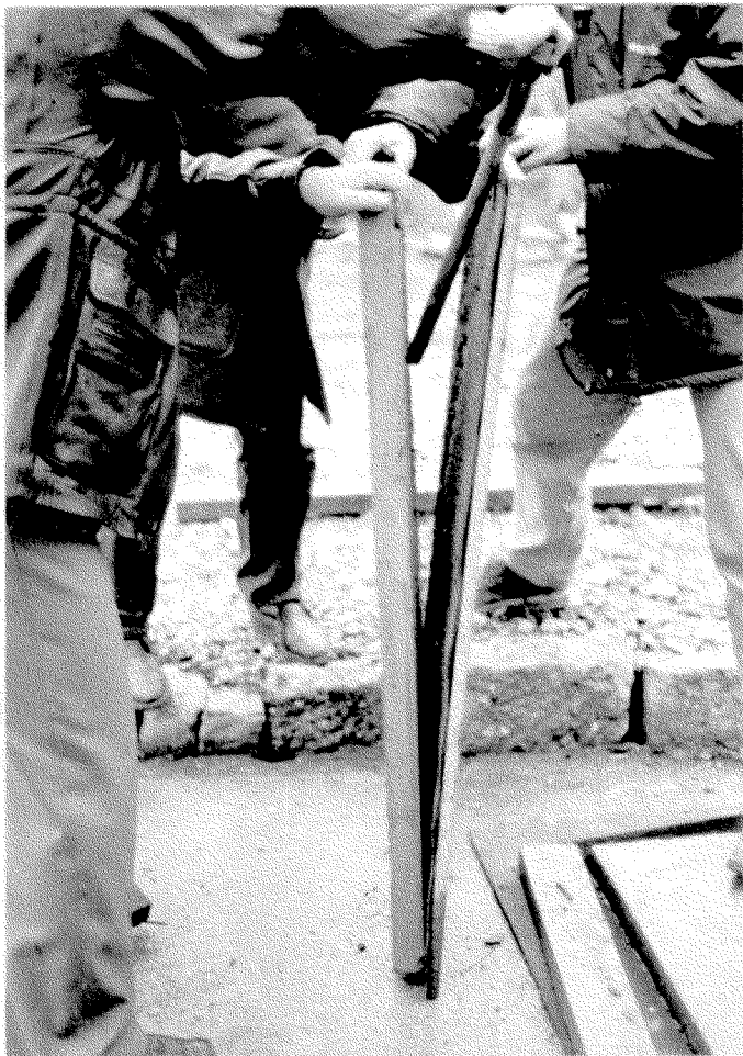
Figure 3 - Prying of the concrete slab
