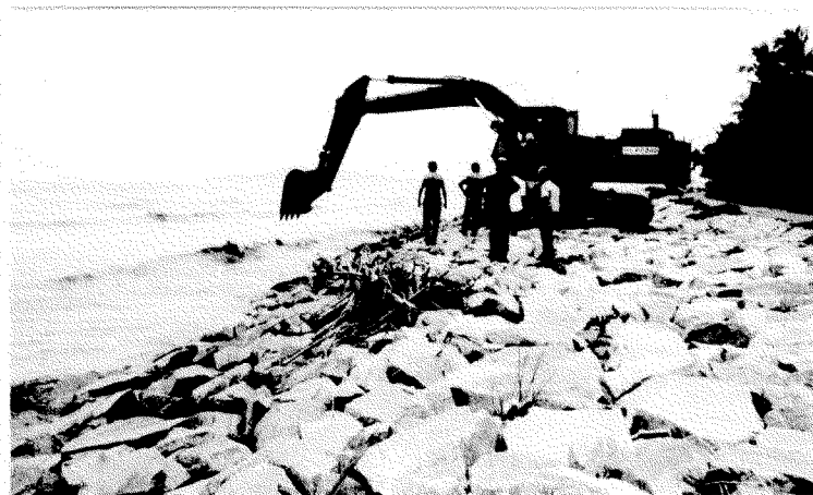
Plate 1. Condition of the revetment before excavation - Site A.
