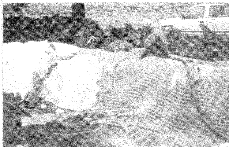
Figure 4 - Arnold Canal test sections 7 through 10. Installation of grout-filled mattress.
