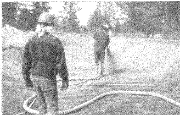
Figure 2 - Arnold Canal test sections 1 and 2. Application of shotcrete cover over geomembrane.
