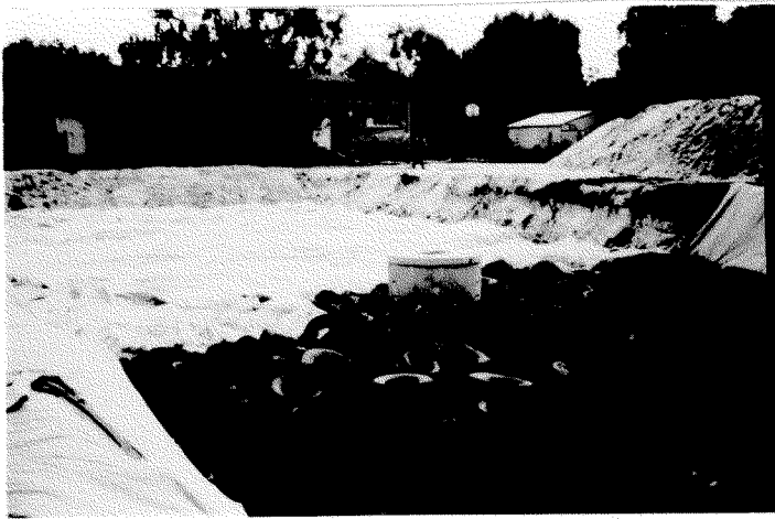
Fig. 1 Geotextile envelope around tyres
