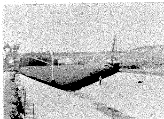
Figure 4 Gravel Cover Material Placement
