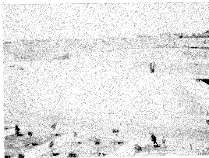
Fig. 2 Regulating reservoir lined with CSPE geomembrane at Agua Prieta
