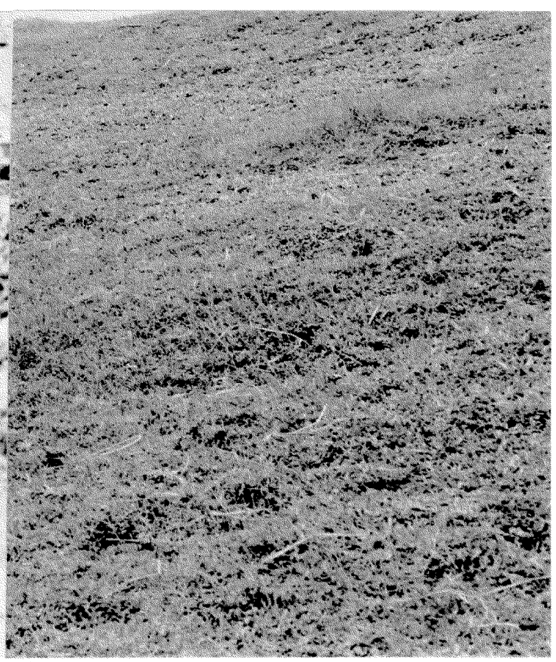
Fig 3. Geojute protected and maintained slope
