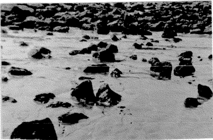
3. 600mm Siltation over the laid Jute Geotextile after a period of 8 months.
