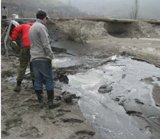
Fig. 7 Filtration of liquid phase of pulp through the screen from nonwoven geotextiles.
