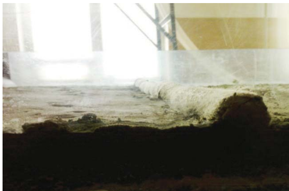
Fig. 4 Sleeve from nonwoven geotextiles filled with tails (in profile)
