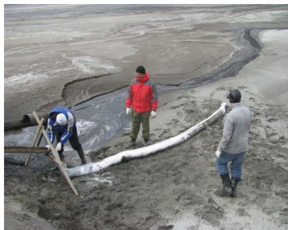
Fig. 6 Filling of sleeve from nonwoven geotextiles with tails by hydromechanization method.
