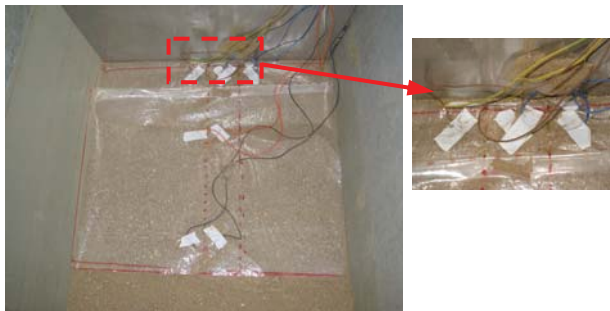
Fig. 11 Geomembrane of SX-3 after operation
