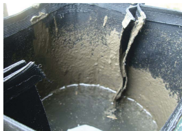
(a) Before backwashing
