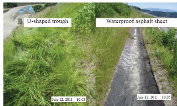
Fig. 16 Weed control effect of berm drains
