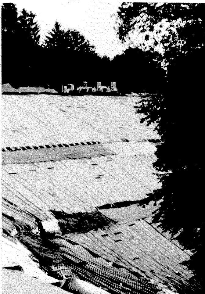
Figure 3 Landfill Covering with an Inclination of 26° (Scheu and Jas, 1992)
