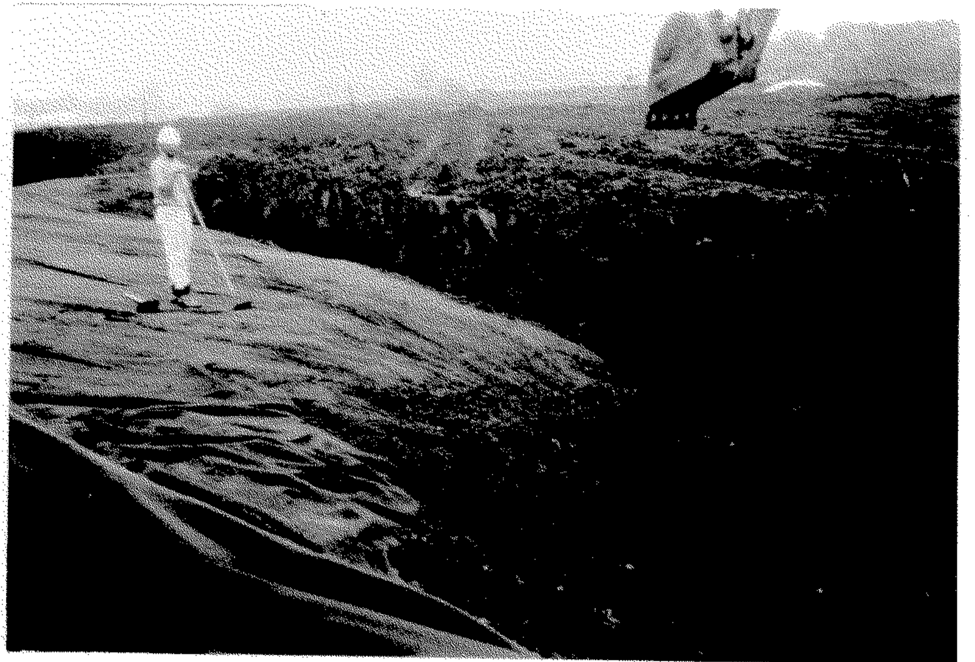
Fig. 4 Removal of cover soil for inspection of geosynthetics for damage or seam separation.
