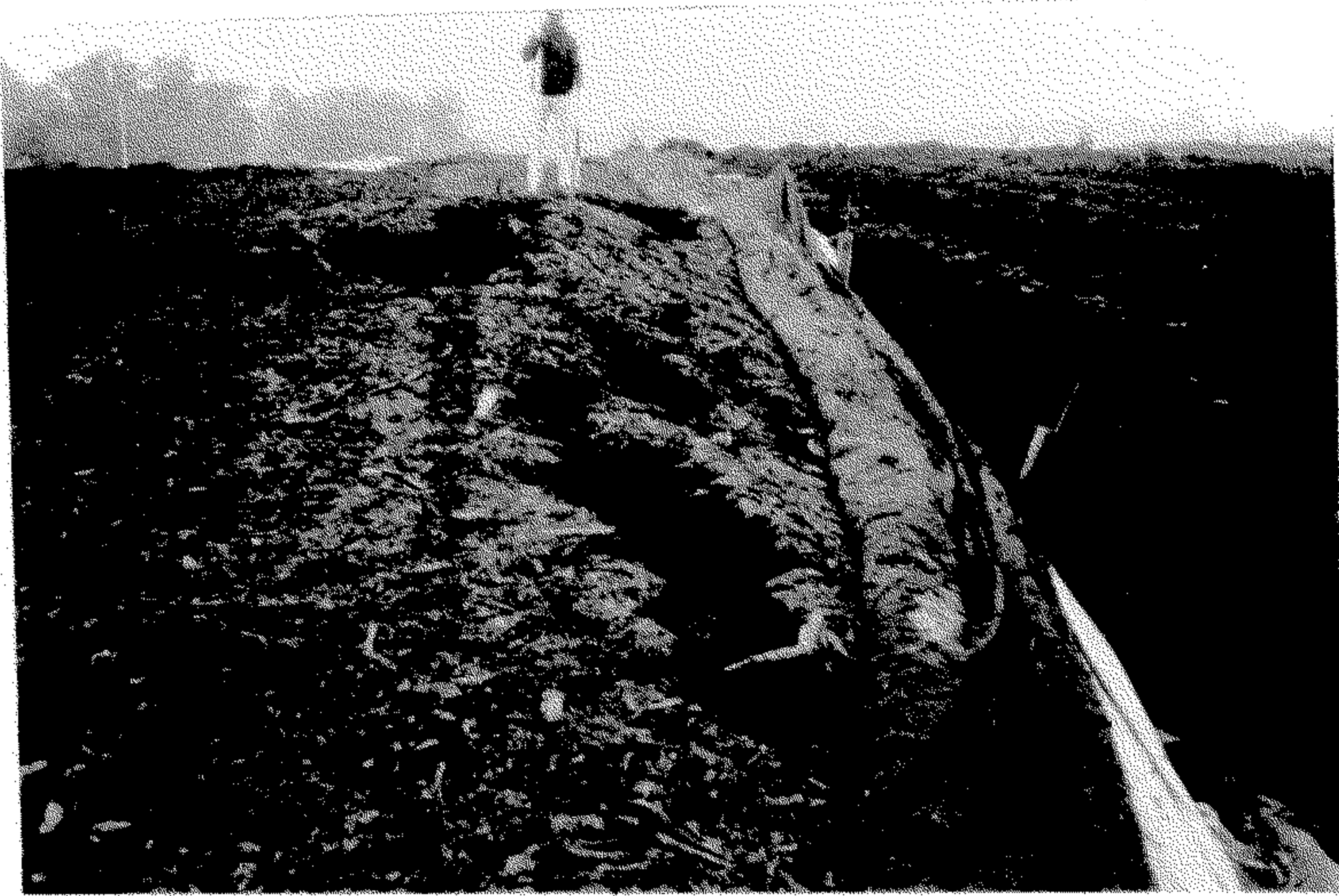
Fig. 2 A view of the localized bearing capacity failure caused by placement of excessive thickness of soil.
