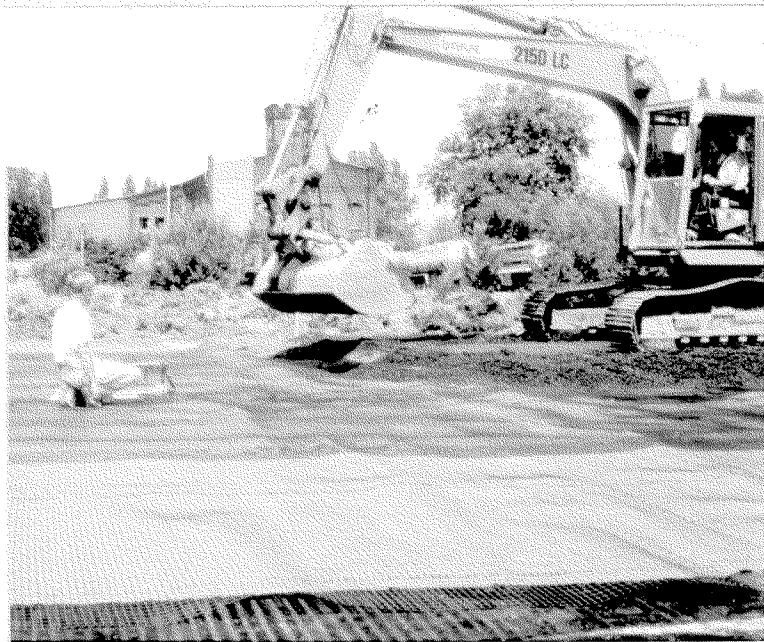
Fig. 3: Placing of geogrids and geomembranes.
